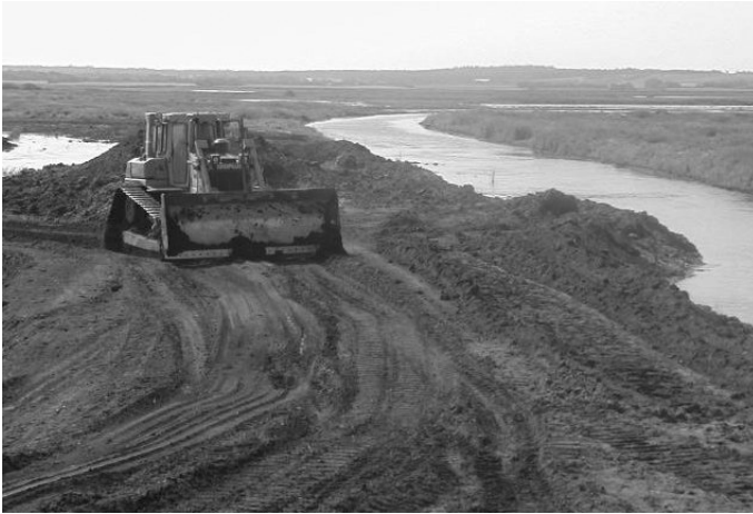
Figure 1.4 A major river restoration project in Europe is being carried out on the Skjern River in Jutland, Denmark, where Denmark’s largest river is being restored to its former meandering course. When the restoration is complete, 2200 ha of meadows and wetlands—half of the area drained in the 1960s—will be restored. A reason for the restoration is coastal pollution in a fjord adjacent to the North Sea caused by the straightened river and pollution transport from agriculture. The Danish public funds earmarked for this project are 8.5 times the cost of the original river drainage project, most of which occurred in the mid-twentieth century. (Photo by W. J. Mitsch.)
