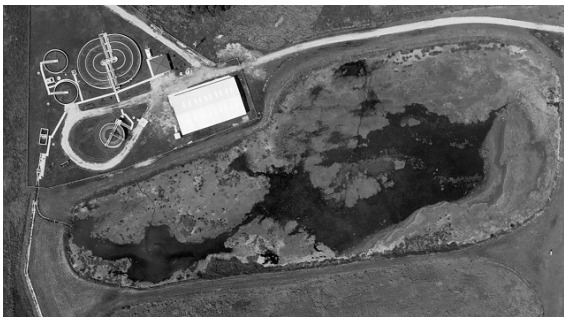
Figure 1.5 A 3-ha treatment wetland adjacent to a wastewater treatment plant in central Ohio. The treatment plant delivers secondarily treated wastewater to the wetland that has, as its main function, tertiary treatment of the wastewater to prevent nitrogen and phosphorus from reaching the adjacent north fork of the Licking River. (Courtesy of W. J. Mitsch.)
