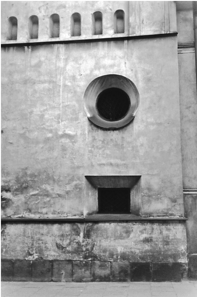
FIGURES 2.14, 2.15 These two buildings in Krakow, Poland, show careful flashing of sills. While both may be remedial, they complement the appearance. The sills, even at the ocular window, of this stuccoed masonry building (Figure 2.14) are flashed in metal. In Figure 2.15, the layers of the wood windowsill have been carefully flashed, with small up-stands or dams at the ends. Photos by Linda Brock.
