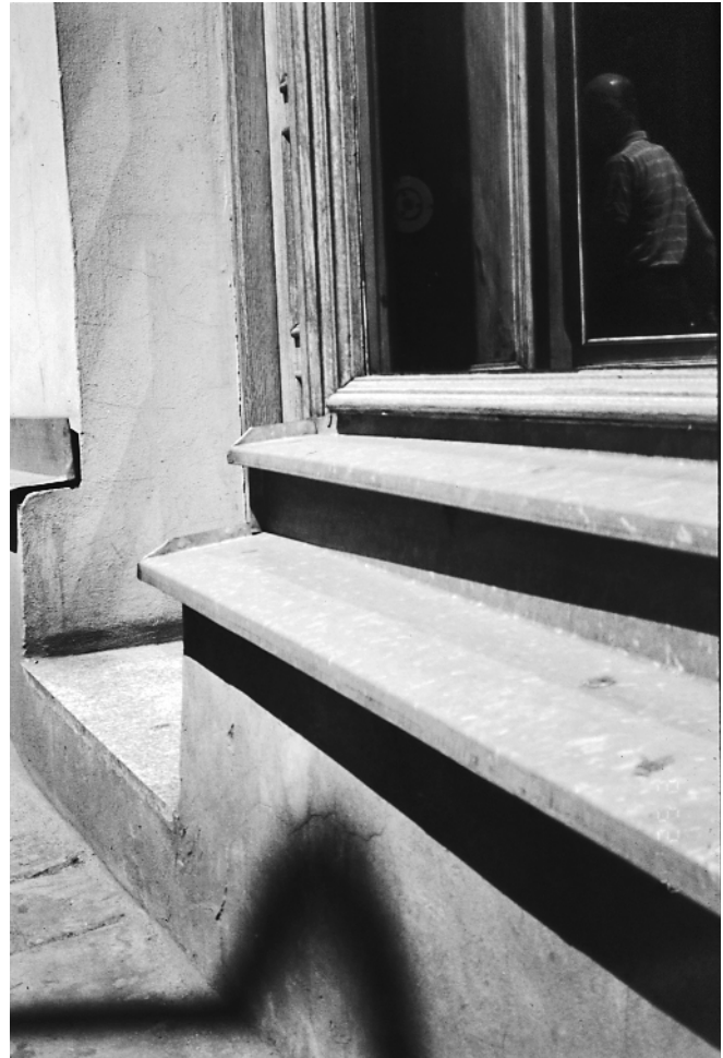
FIGURES 2.14, 2.15 These two buildings in Krakow, Poland, show careful flashing of sills. While both may be remedial, they complement the appearance. The sills, even at the ocular window, of this stuccoed masonry building (Figure 2.14) are flashed in metal. In Figure 2.15, the layers of the wood windowsill have been carefully flashed, with small up-stands or dams at the ends. Photos by Linda Brock.
