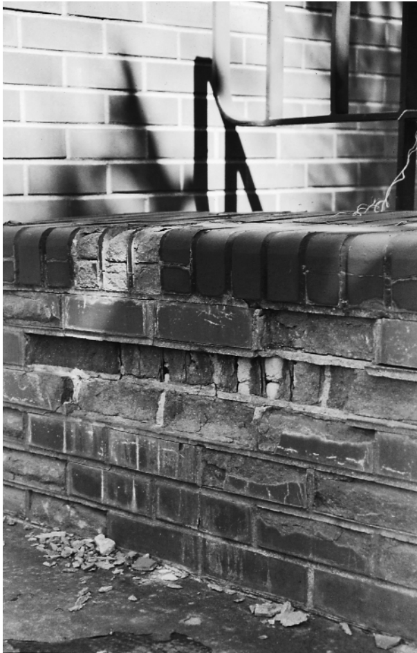
FIGURES 2.8, 2.9 These photographs show conditions on a building when it was approximately 14 years old. It is located in an area that receives about 19 inches (480 mm) of precipitation a year. The bench (Figure 2.8), located on a bridge that connects two wings of the building and the parapet (Figure 2.9), were waterproofed with an elastomeric coating. When water entered the walls through the inevitable cracks and pinholes, it could not get back out. Freeze-thaw action exacerbated the damage. Photos by G. Russell Heliker.
