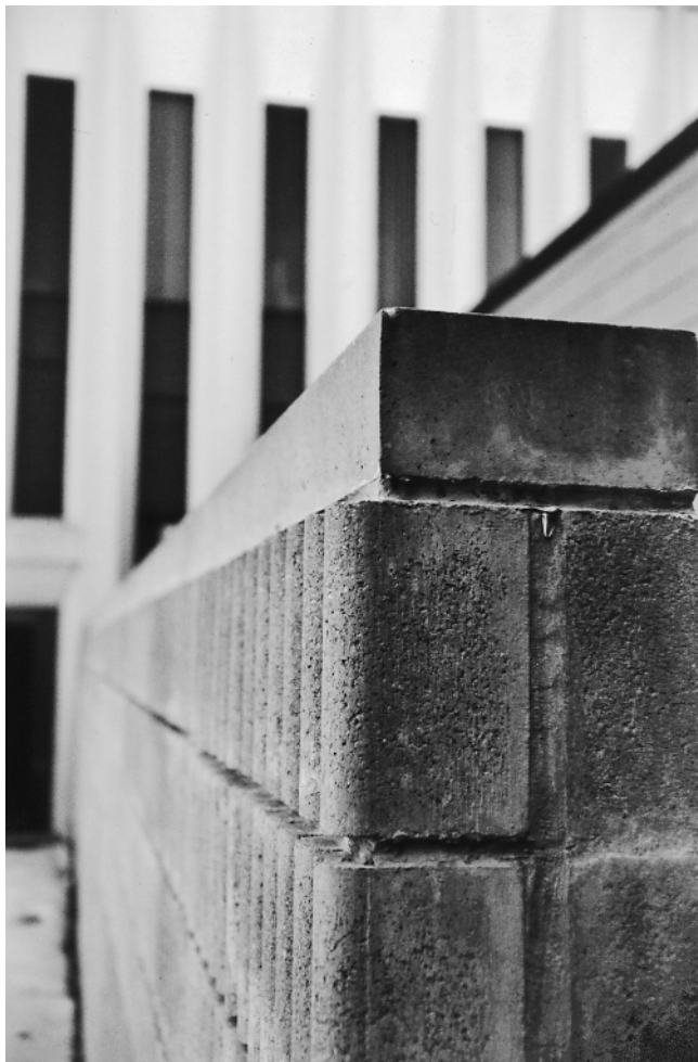
FIGURES 2.12, 2.13 The top of this parapet wall (Figure 2.12) was detailed by the architect with a decorative concrete block course. Aesthetically interesting, it leaked considerably. The owners retrofitted the metal flashing (Figure 2.13), which did a good job of keeping out the water, but the aesthetic was changed. Photos by G. Russell Heliker.
