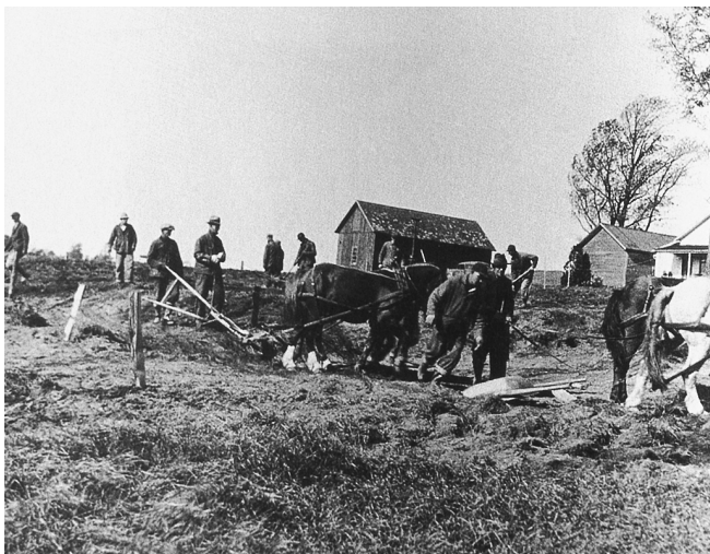
Figure 1-5 Before the era of the internal combustion engine and powerful earthmovers, horses and men built golf courses with rather crude tools.
