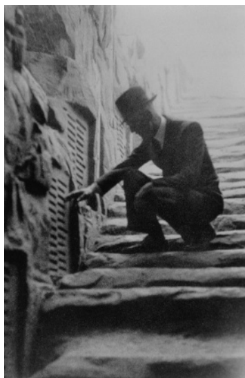
FIG. 3.14 This Nilometer was carved into rock on the shore of the Nile River near Aswan, Egypt. During ancient times, Nilometers were used to determine taxes as well as the proper time to break dikes to begin irrigation of fields.
