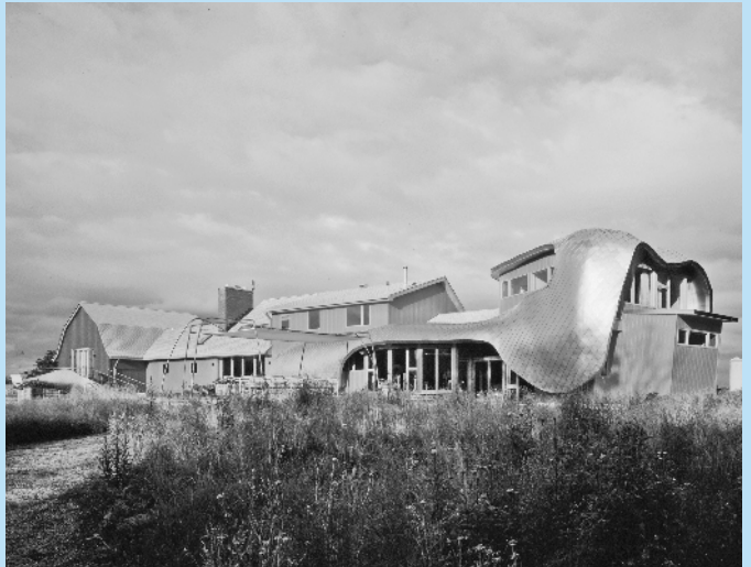
Spring Prairie Residence, Spring Prairie, Wisconsin. Architect: Garofalo Architects. Photographer: Nathan Kirkman.
