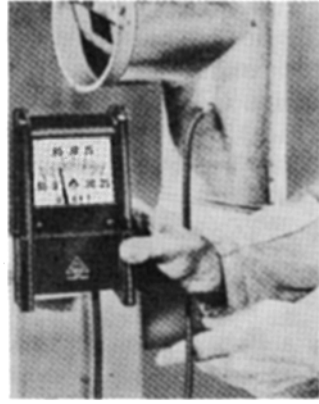
(B) Flue pipe draft.
