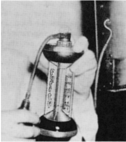
Figure I-43 Bacharach Fyrite CO 2 indicator.
