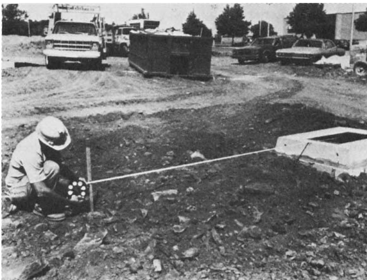
Figure I-1 One way of laying out is with a hundred-foot tape. Metal tape is standard, but this new fiberglass one works well and cleans easily. (Courtesy of Stanley Tools.)
