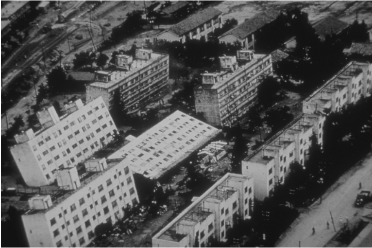
Figure 1.7 Liquefaction-induced damage. Image of leaning apartment houses following Niigata Earthquake, Japan 1964. Reproduced from http://www.ngdc.noaa.gov/seg/hazard/slideset/1/1_25_slide.shtml 01/06/08 by permission of the National Geophysical Data Center.
