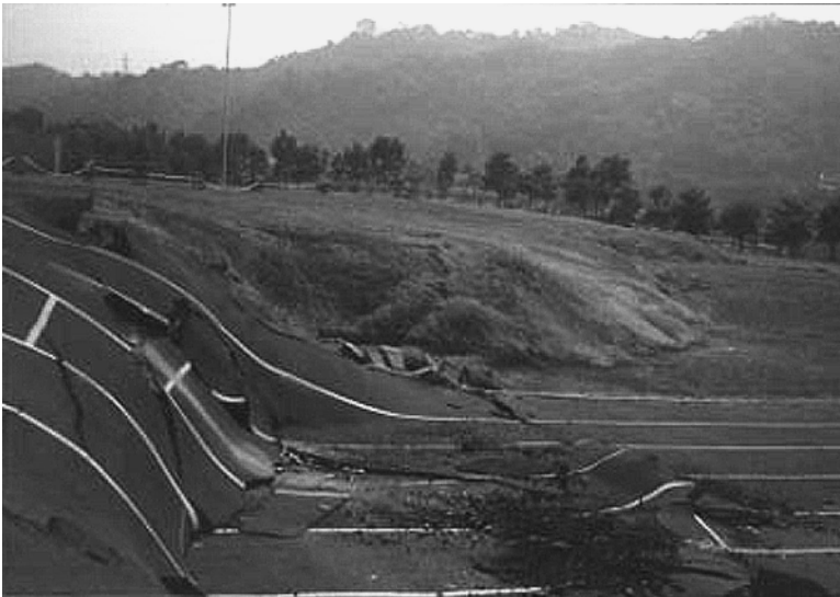
Figure 1.8 Subsidence of a running track by more than three metres. Reproduced from http://www.whfreeman.com/bolt/content/bt00/figure2.jpg 08/04/08 by kind permission of Beverley Bolt.
