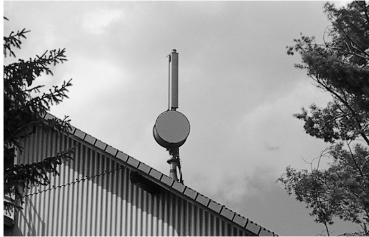
Figure 1.18 A typical antenna of a GSM base station. The optional microwave directional antenna (round antenna at the bottom of the mast) connects the base station with the GSM network
