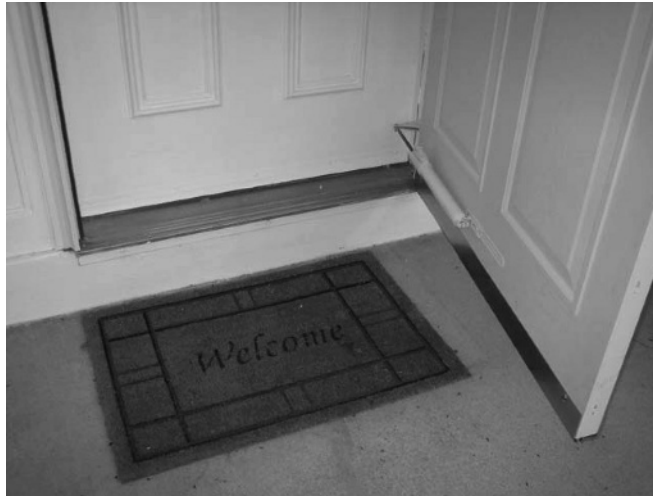
Figure 1.2 An EMCO screen door hinge, lower, where more people can reach it.
