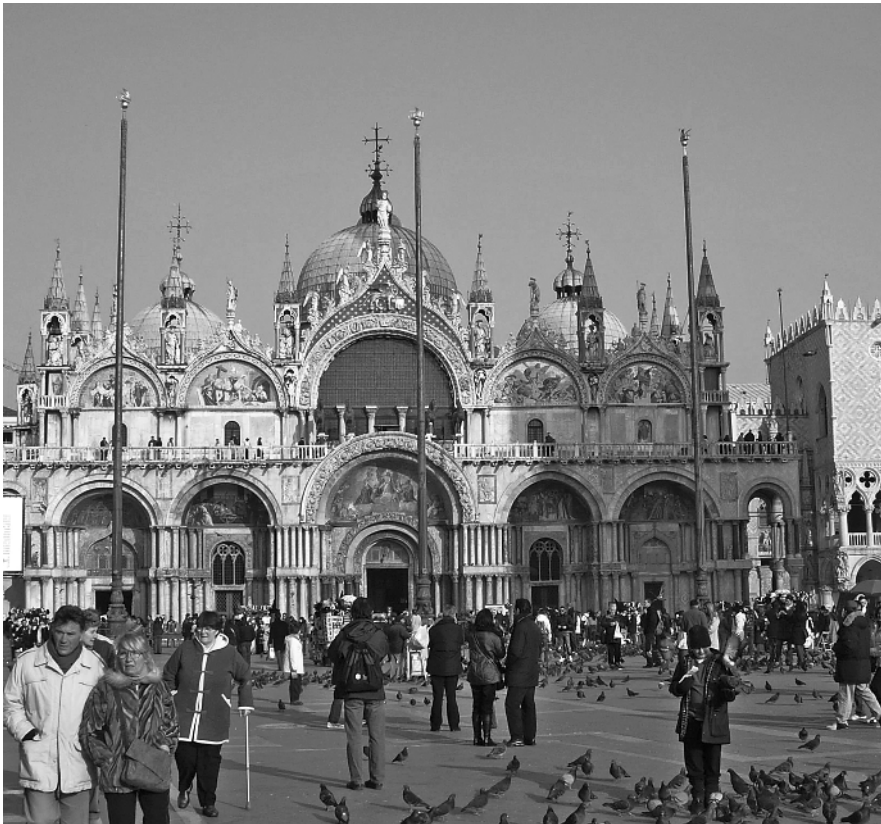
Photo 1.1 Basilica of S Marco, Venice, c 830 (rebuilt 11th century). Reflecting Venetian trading importance, Europe's most flamboyant cathedral combines Byzantine and western styles. With its Greek cross plan, large central dome and smaller domes over the aisles and transepts, the edifice is the focal point of the Piazza S Marco.
