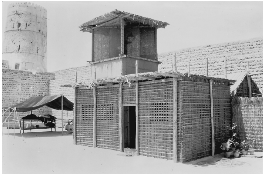
Figure 1.2d When additional ventilation is desired, wind scoops can be used, as on this reconstructed historical dwelling in Dubai. Also note the open weave of the walls to further increase natural ventilation. (Photograph by Richard Millman.)
