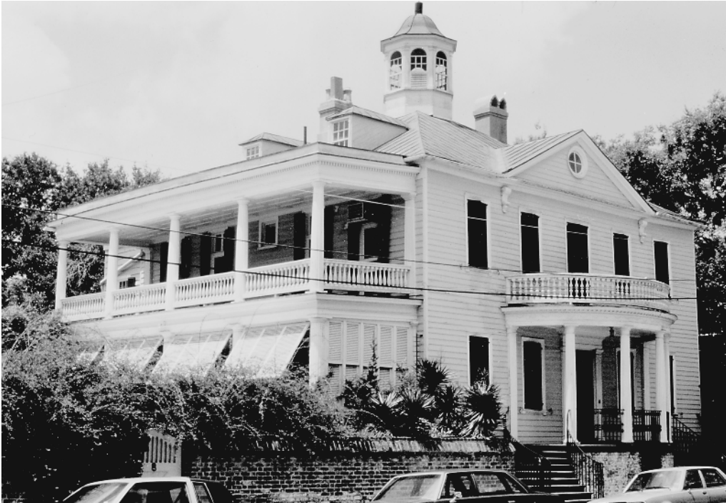
Figure 1.2b In hot and humid climates, natural ventilation from shaded windows is the key to thermal comfort. This Charleston, South Carolina, house uses covered porches and balconies to shade the windows, as well as to create cool outdoor living spaces. The white color and roof monitor are also important in minimizing summer overheating.
