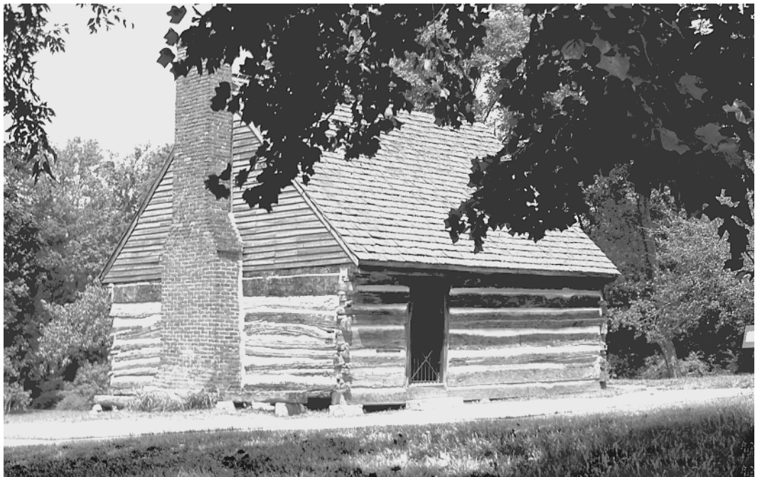
Figure 1.2f In cold climates, compactness, thick wooden walls, and a severe limit on window area were the traditional ways to stay warm. In very cold climates, the fireplace was located either on the inside of the exterior wall or in the center of the building.
