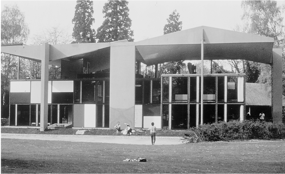
Figure 1.3g The “Maison d’Homme” in Zurich, Switzerland, demonstrates well the concept of the parasol roof. The building is now called “Centre le Corbusier.” (Photograph by William Gwinn.)
