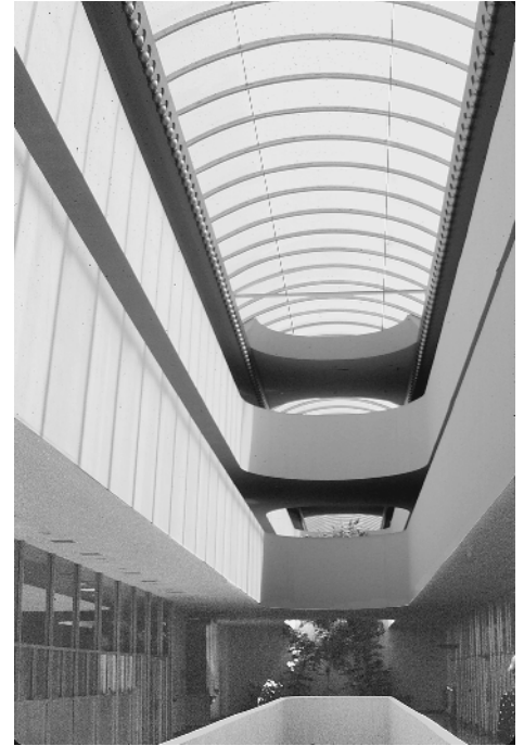
Figure 1.3e In the linear central atrium of the Marin County House, F.L. Wright used white surfaces to reflect light down to the lower levels. The offices facing the atrium have all-glass walls.
