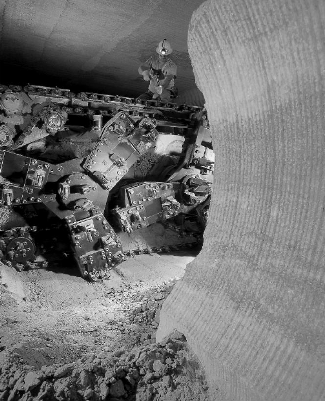
FIGURE 1-2 A mechanic making repairs and adjustments to the front end of a continuous boring machine in potash service.
