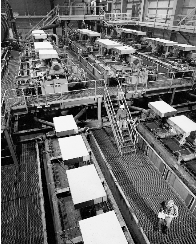
FIGURE 1-15 Banks of flotation cells used for the production of potash concentrate.
