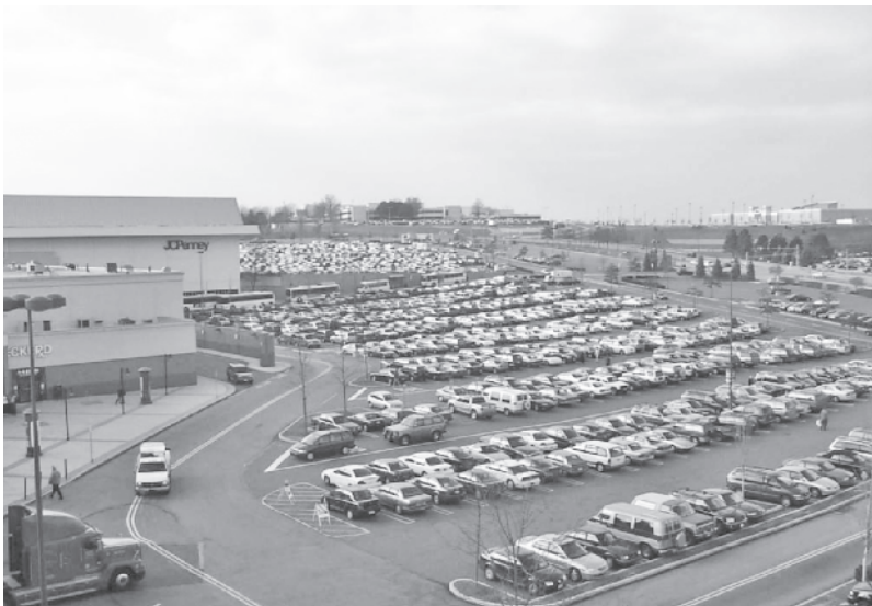
Figure 1-13 A typical commercial site, with the building surrounded by a sea of impervious pavement.
