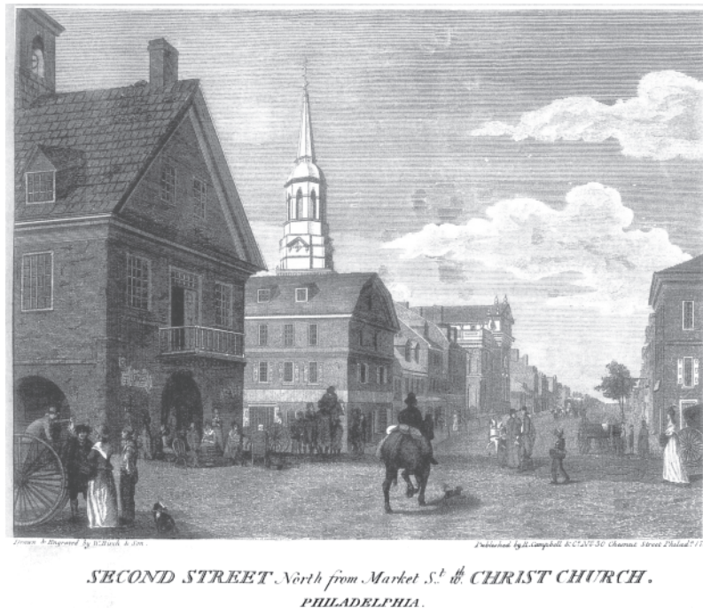
Figure 1-11 The urban environment in the eighteenth century (1799). The road was pervious.
