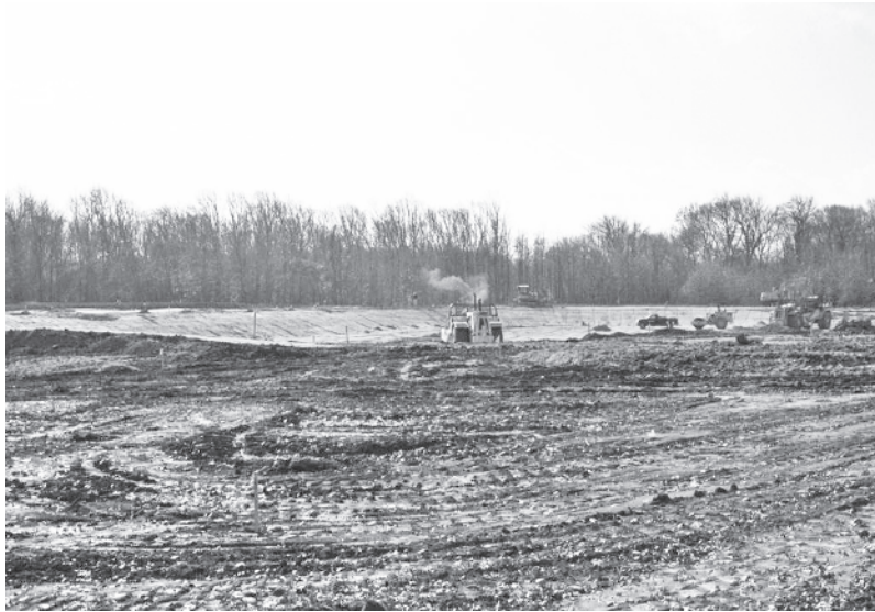
Figure 1-22 Detention basin construction removes vegetation and compacts the soil, reducing infiltration and evapotranspiration.
