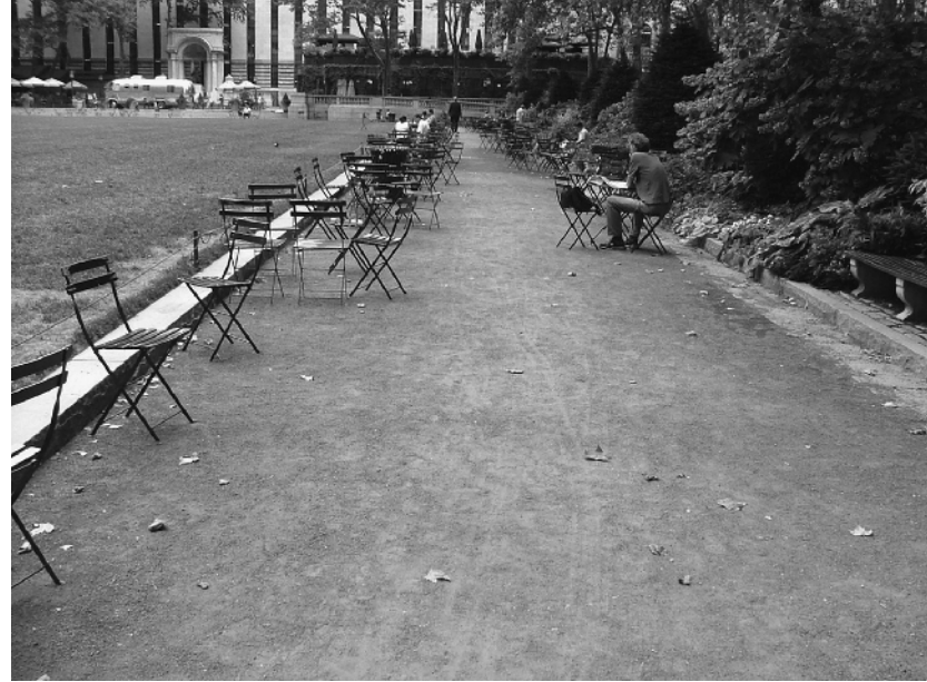
Figure 1-6 This aggregate walkway endures intense urban foot traffic while providing adequate support for the narrow legs of the site furnishings.
