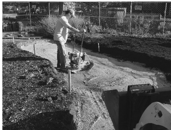
Figure 1-5 Adequate leveling and compaction are critical when aggregate is used as a base course supporting other paving materials.
