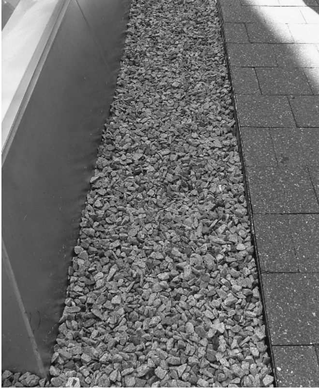
Figure 1-2 This aggregate installation serves as an economical, low-maintenance solution for good drainage along the foundation wall of a building.
