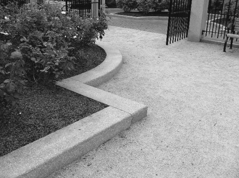
Figure 1-4 A well-compacted ungraded aggregate surface provides a stable and visually appealing walking surface at a far lower cost than concrete, asphalt, or masonry unit pavers.
