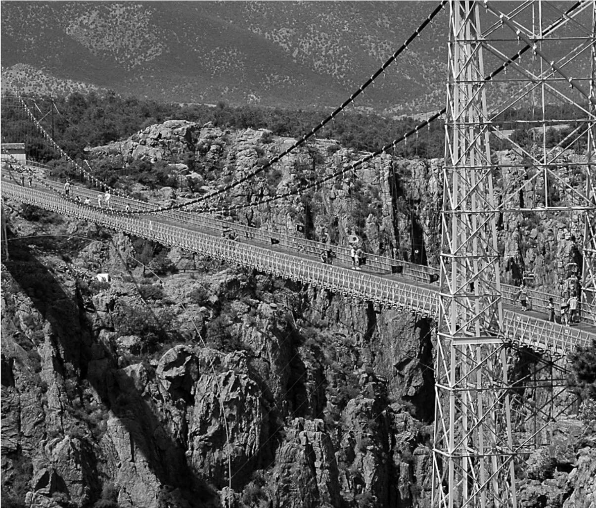
**Figure 1.43** The Royal Gorge Suspension Bridge, designed by George Cole and constructed in 1929, spans 268.2 m (880 ft) over the Arkansas River in Colorado. The river lies 321 m (1,053 ft) below. Two dramatic funicular cables pull both down and out on the deck to stabilize the narrow bridge. One is visible as a white arc to the lower left.
