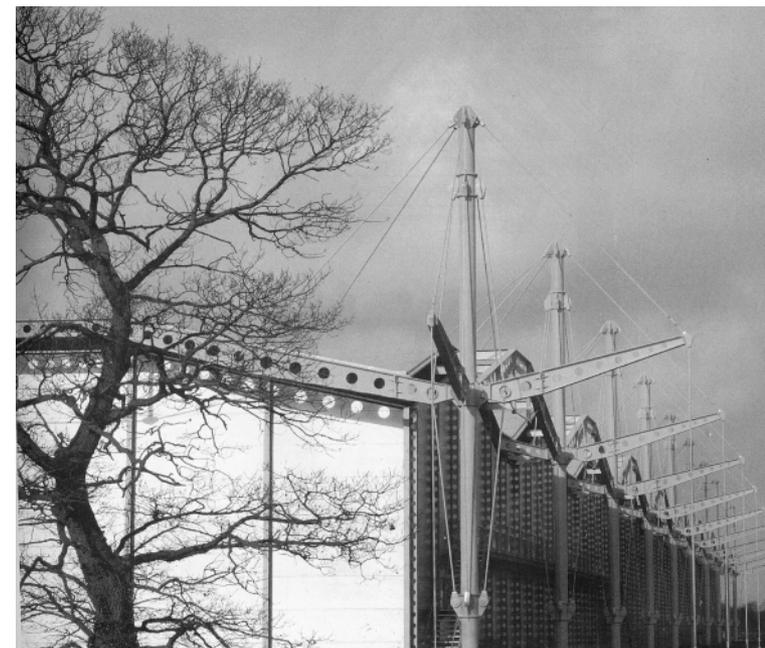
**Figure 1.46** The roof of the Renault Centre at Swindon, England, is supported by an ingenious arrangement of steel rods and beams. (Architect: Norman Foster. Structural engineer: Arup Associates.)
