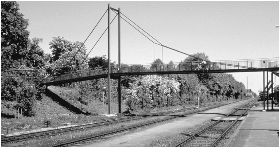
◄ **Figure 1.51** Schlaich Bergermann collaborated in 1988 with architect Eberhard Schunck to use funicular rods to support a pedestrian bridge over the railroad tracks at Bad Windsheim in Germany.
