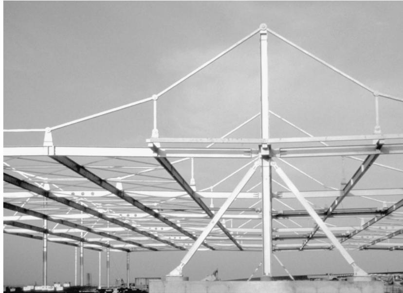
◀ **Figure 1.52** The engineers at Schlaich Bergemann used a similar arrangement of rods to suspend this large-span factory roof at Dachwig, Germany, providing an efficient solution and eye-catching profile to satisfy the client's desire for corporate identity. It is shown here during construction in 1993.
