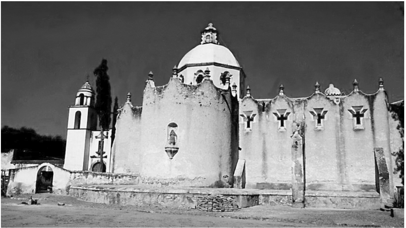
▲ Figure 1-7 Restored exterior of the church of Jesús Nazareno in Atotonilco in north central Mexico, which in the 1990s suffered extensively from both rising damp and roof water leakage.
