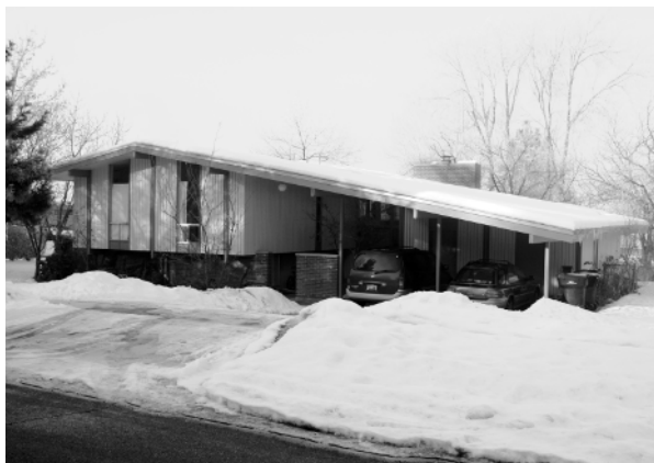
Figure 1.7 Systematized onsite building construction was developed in the mid-twentieth century and continues today as the pervasive method of residential construction. This house in Utah is modeled after mid-century Eichler houses. There are neighborhoods throughout the western United States that are built within the principles of courtyards, large expanses of glass set within a post-and-beam structure.
