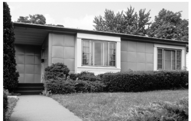
Figure 1.6 The 1948 Lustron House was an all-enamelled steel building system that used the automobile metal sandwich panel technology. This Lustron home still stands in Madison, Wisconsin.
