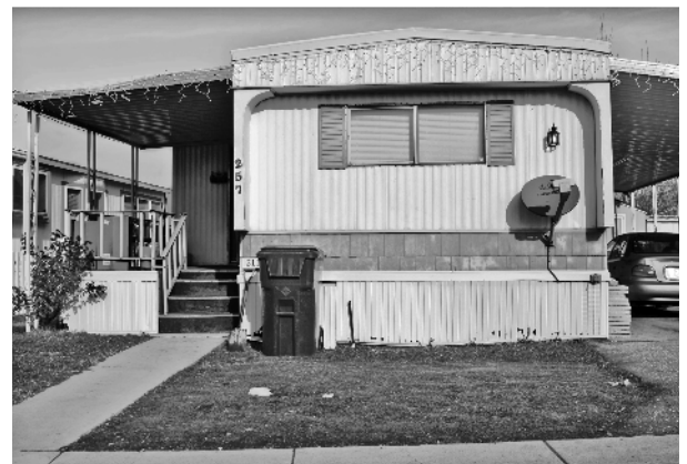
Figure 1.8 A late 1970s single-wide mobile house with flanking porches near Salt Lake City, Utah, built to HUD code.
