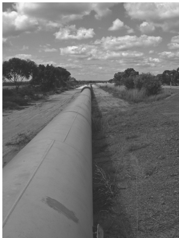
Figure 1.8 A pipeline in the Goldfields Water Supply Scheme, Perth, Australia (Source: http://en.wikipedia.org/wiki/Image:Goldfields_Pipeline_SMC.JPG ).
