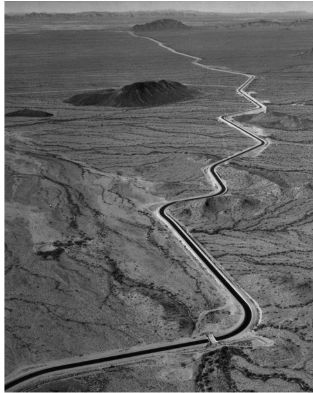
Figure 1.6 Central Arizona Project aqueduct (Source: http://en.wikipedia.org/wiki/Image:Arizona_cap_canal.jpg ).
