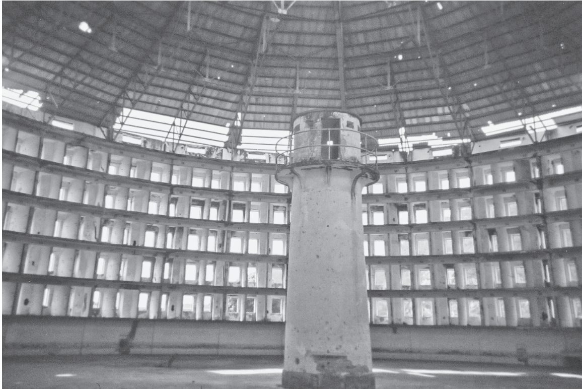
Figure 1–6: The Panopticon. Developed by Jeremy Bentham, an English natural philosopher, the Panopticon is a design concept for prisons that, in its purest form, allows the guards, stationed in the middle of a circular plan, to have direct surveillance of all prisoners, whose cells are arrayed around the perimeter of the circular plan and stacked on multiple floors. Due to the configuration, prisoners cannot see into nearby cells.
