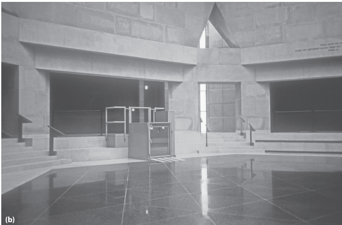
Figure 1-11: Hall of Remembrance at the Holocaust Memorial in Washington, DC. (a) Stairs surround the main floor level of the Hall. (b) A mechanical lift is installed on the stairs to provide access to the lower level.
