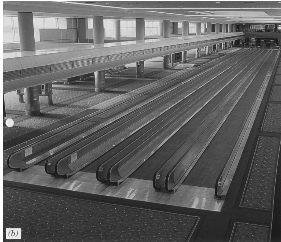
Figure 1.13. Moving walkways: (a) inclined, (b) flat (Courtesy KONE).
