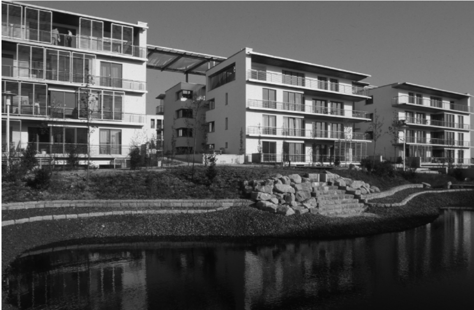
◀ At Kronsberg, a sustainable, mixed-use community in Hanover, Germany, storm water is collected in ponds. In the background, a residential building has movable sunscreens to control heat gain. Willen Associates Architekten. Photo by Karl Johaentges.
