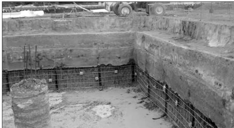
Figure 1.26 Shotcrete and helical anchor shoring system
