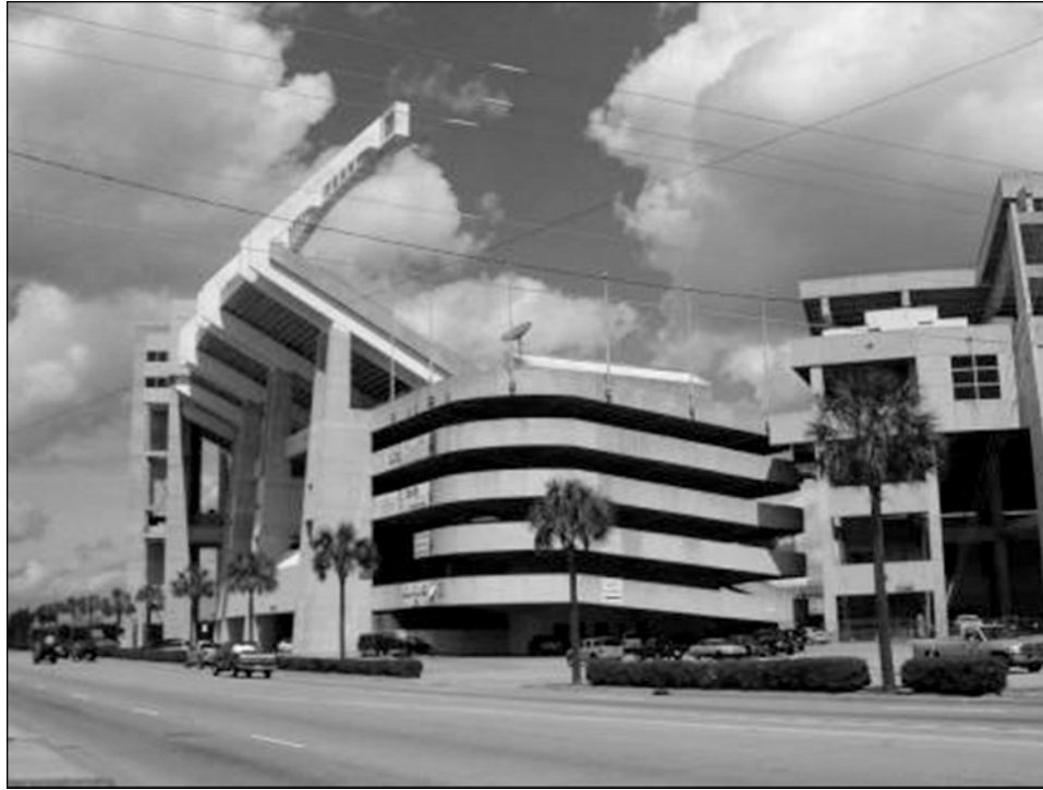
Figure 1.22 Stadium locker room addition
