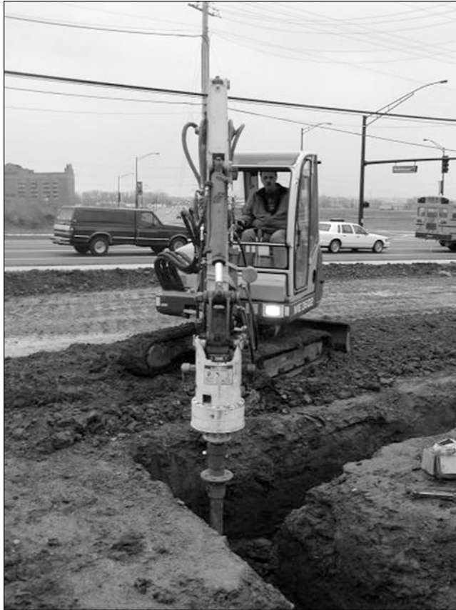
Figure 1.24 Adverse weather installation (Courtesy of Magnum Piering, Inc.)
