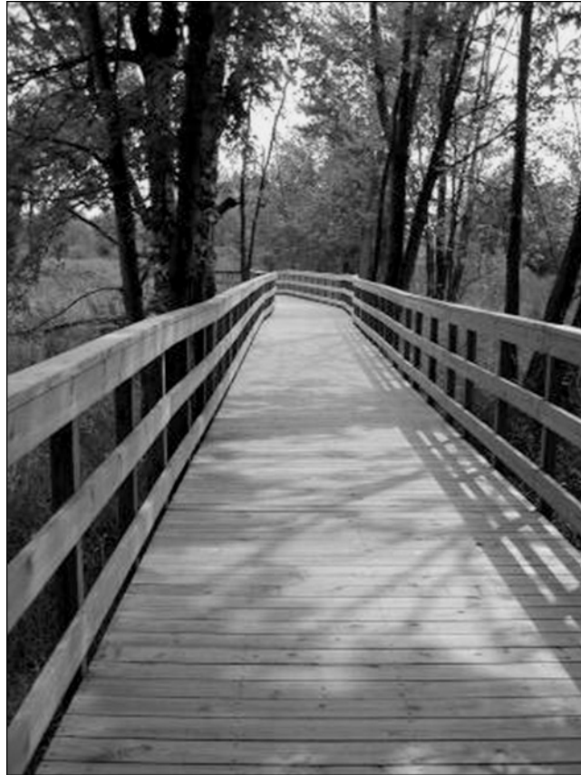
Figure 1.21 Nature walk construction (Courtesy of Magnum Piering, Inc.)
