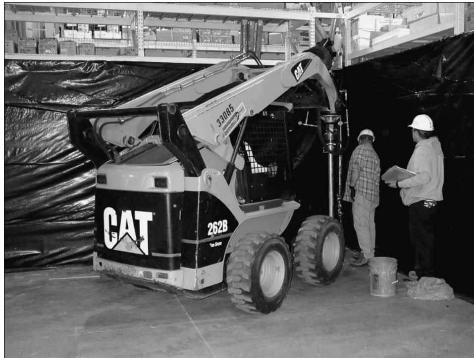
Figure 1.23 New mezzanine foundation (Courtesy of Earth Contact Products, Inc.)
