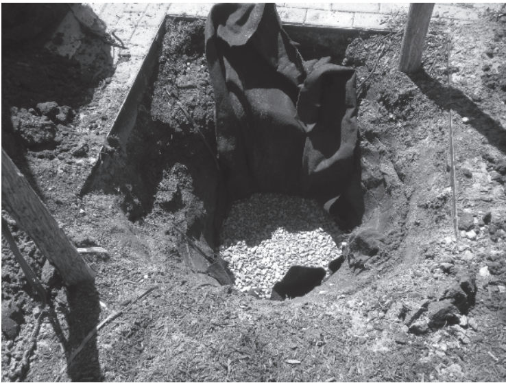
Figure 1.25 After determining the water level, place a layer of stone on a geotextile fabric to elevate the root ball so that it is sitting above the water level.
