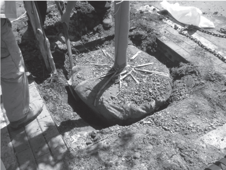
Figure 1.26 The root ball is set on the stone with the tree flare slightly above the surrounding grade, keeping the root ball as high as possible.
