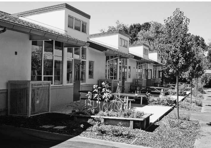
New light monitors added during a modernization at Almond School emphasize doors, bring in daylight, ventilate, and introduce better scale and rhythm along the building face. Source: Gelfand Partners Architects
