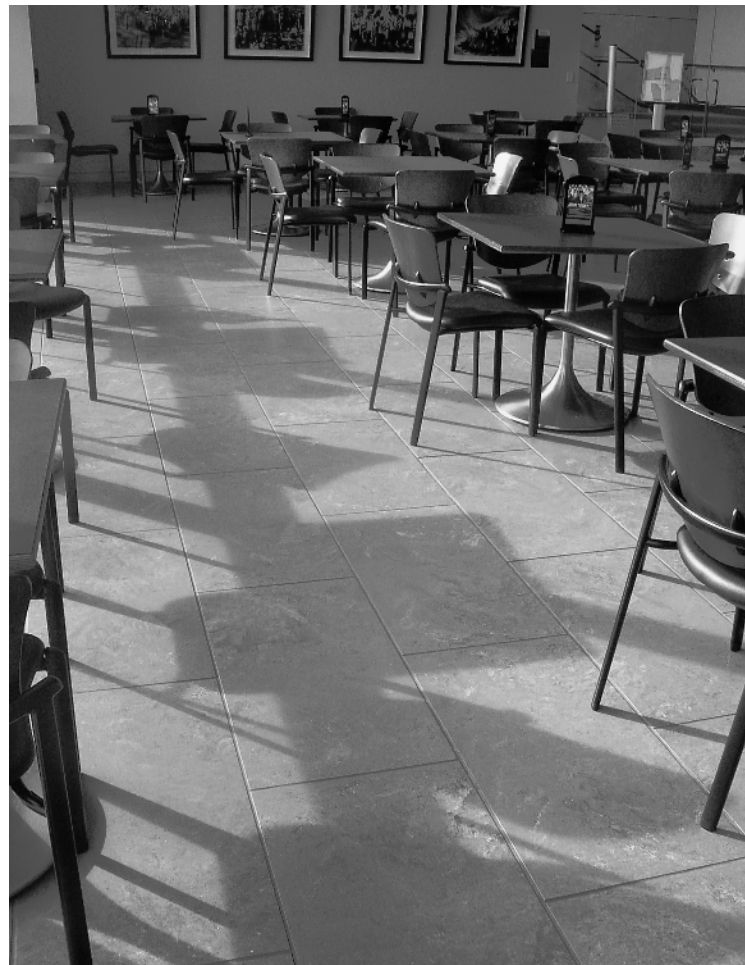
Figure 1-48 Because porcelain tiles are dimensionally stable, narrow grouts and relatively large tiles can be specified and installed. Photography by Bethany Tozar of Impulse Photography.
