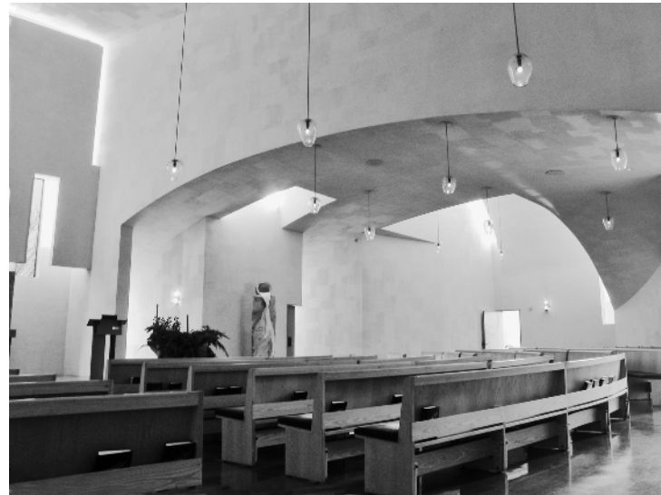
Figure 1-19 The combed surface treatment of the plaster walls and ceiling surfaces in the Chapel of St. Ignatius, Seattle, Washington, is highlighted by indirect, color-tinted daylight. Designed by Steven Holl (1999). Photography by Michael Zaretsky.
