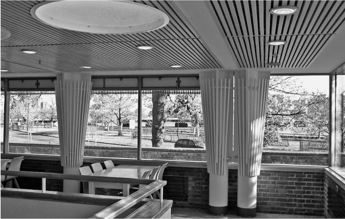
Figure 1-39 The spacing of birch wood slats of the interior millwork helps to improve the acoustics in the dining area of Baker House, Massachusetts Institute of Technology, Cambridge, Massachusetts, designed by Alvar Aalto (1947–1948). Photography by Ben Meyer.
