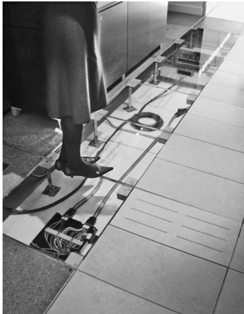
Figure 1-54 TecCrete raised access floor system with Power Base AI, manufactured by Haworth. Photography by Jim Postell.
