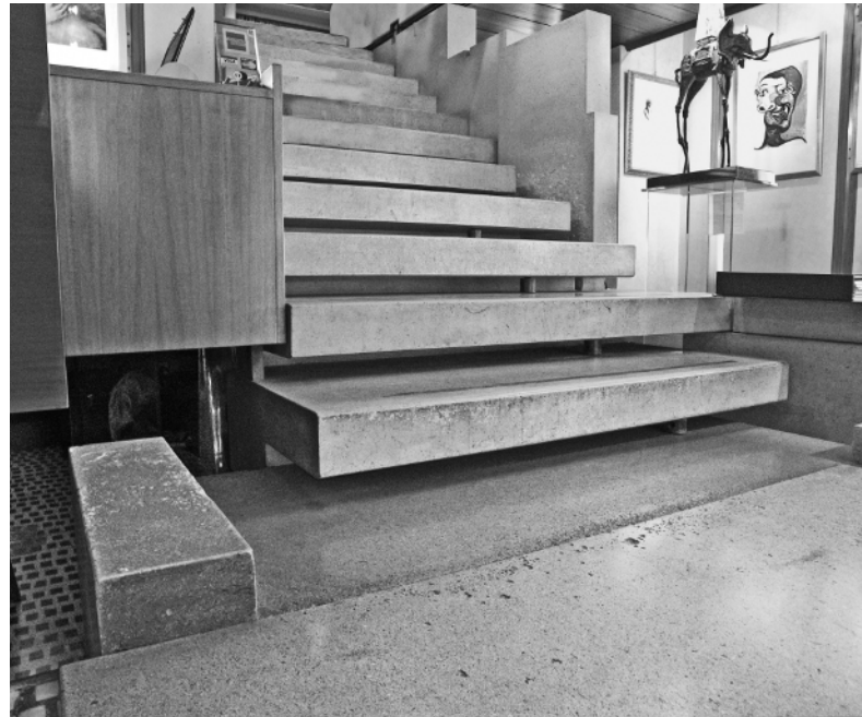
Figure 1-37 Olivetti showroom, Venice, Italy, designed by Carlo Scarpa (1957). Scarpa used concrete to create an interior landscape rich in detail and level changes, to accommodate the periodic flooding that occurs in Venice. Photography by Paul Fatkins.
