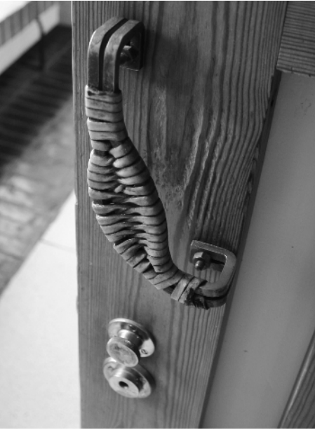
Figure 1-22 Leather-wrapped door handle at Säynätsalo Town Hall, Säynätsalo, Finland, designed by Alvar Aalto (1949-1952). Photography by Jim Postell.
