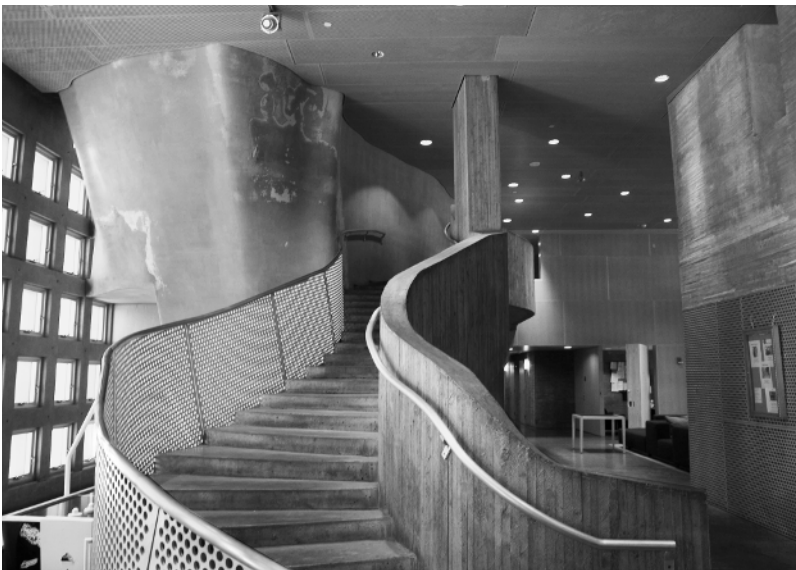
Figure 1-28 Cast-in-place concrete partitions, metal handrails, and wood ceiling, all conventional materials, used in unique ways. Simmons Hall, Massachusetts Institute of Technology, Cambridge, Massachusetts, designed by Steven Holl (1999–2002). Photography by David M. O’Connell.
