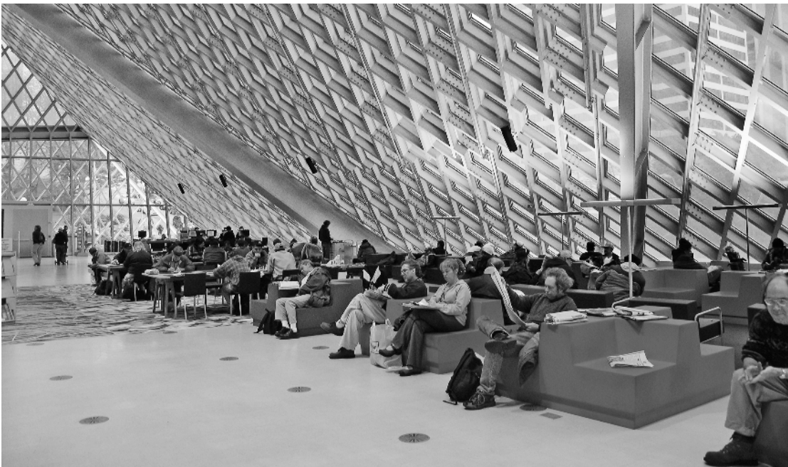
Figure 1-40 In the lobby of the Seattle Public Library, Seattle, Washington, over half of the glass and aluminum curtain walls is triple-pane glazing with an expanded aluminum metal mesh sandwiched between the outer panes. Designed by Rem Koolhaas of OMA (2004). Photography by Michael Zaretsky.
