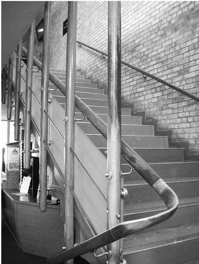
Figure 1-10 The profile of the smooth wooden handrail complements the coarse brickwork at the First Christian Church, Columbus, Indiana, designed by Eliel Saarinen (1940–1942). Photography by Jim Postell.
