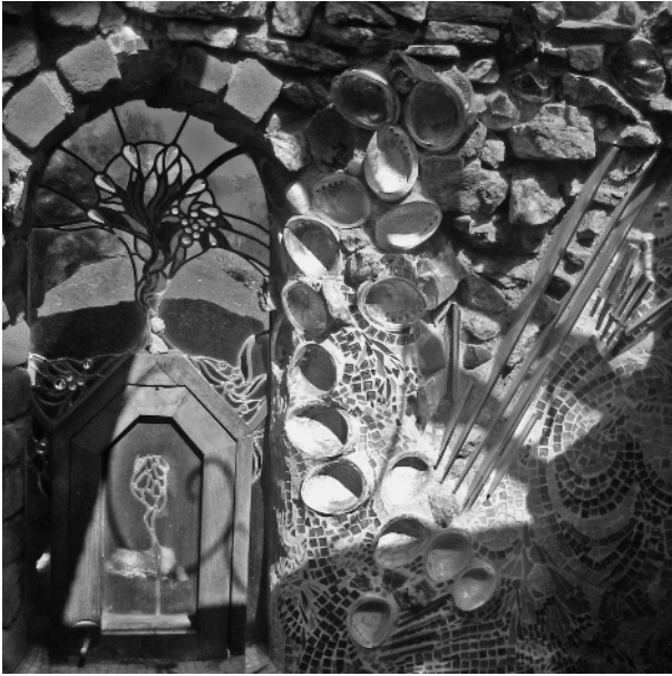
Figure 1-27 Close-up detail of local materials used at the Hubbell residence, Santa Ysabel, California. The hand-formed clay tiles, shells, and broken-glass mosaic are embedded into concrete. Photography by Peter Hilligoss.
