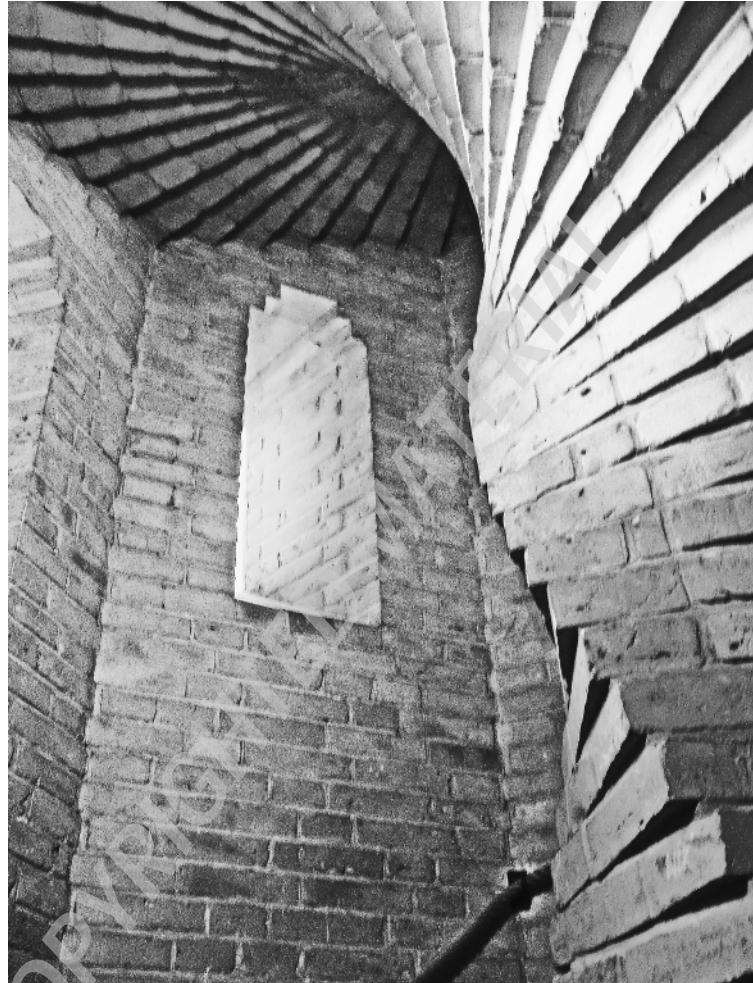
Figure 1-1 Peder Vilhelm Jensen-Klint's stairwell design of Grundtvigs Kirke in Copenhagen, Denmark (1913), intentionally uses whole brick masonry units throughout in order to draw associations between the integrity of the material and the church community. Photography by Sarah Sokoloski.
