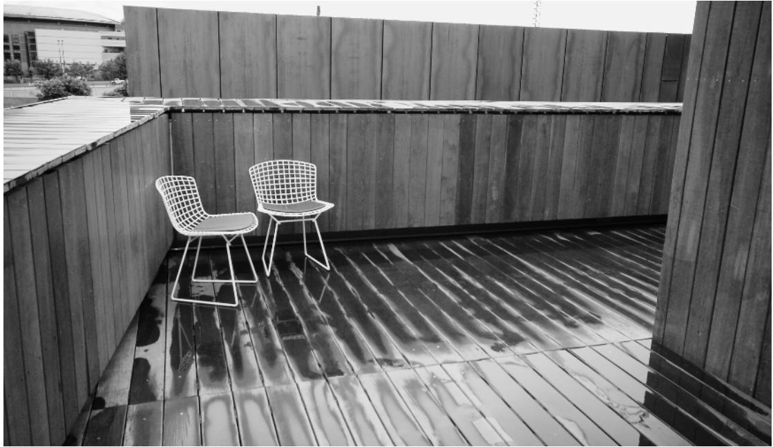
Figure 1-45 ¾-inch ipe lumber used for outdoor decking and guardrail parapet at the Museum of Contemporary Art, Denver, Colorado, designed by David Adjaye (2009). The building is Gold LEED certified. Photography by Malcolm Lee.
