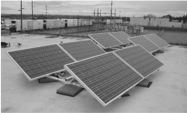
Figure 1.2. Two-kilowatt PV array from JX Crystals Inc on a commercial building flat rooftop.
