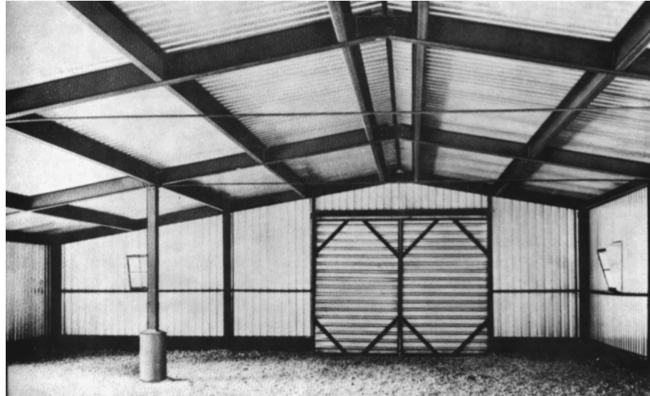
Figure 1.20 Small building made entirely of cold-formed sections. (Courtesy of Stran-Steel Corporation.) 1,6
