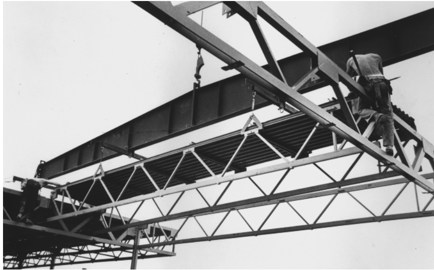
Figure 1.17 Steel deck is designed as the top chord of prefabricated open web steel joists. (Courtesy of Inland-Ryerson Construction Products Company.)
