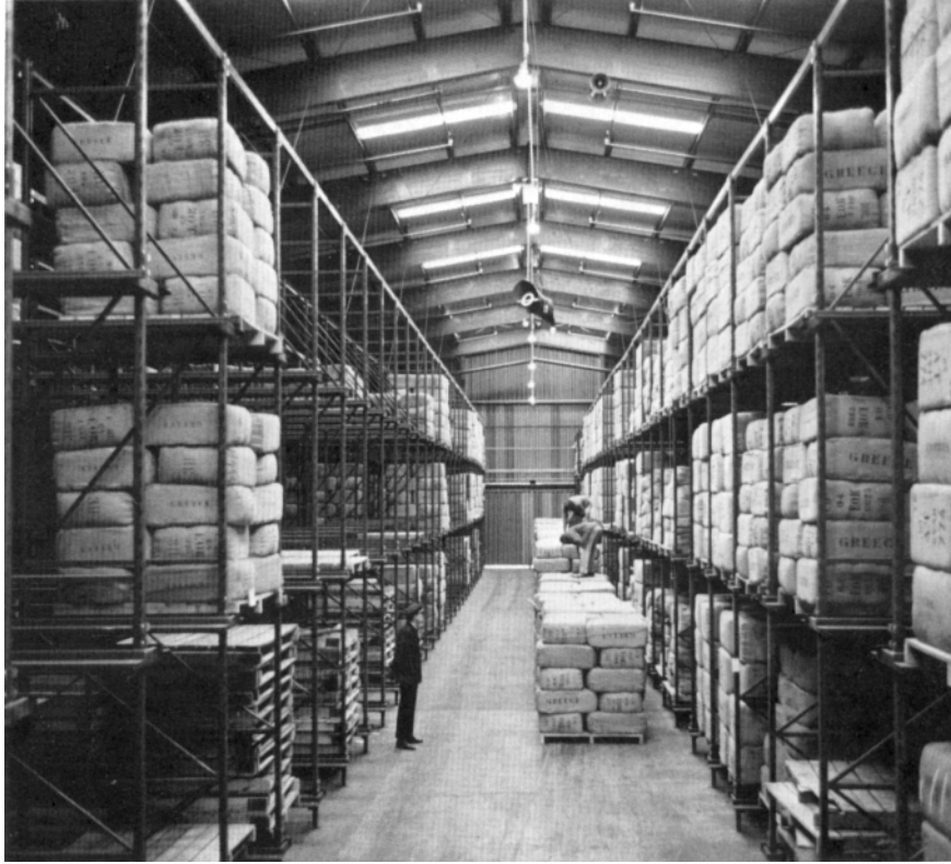
Figure 1.10 Rack structures. (Courtesy of Unarco Materials Storage.)
