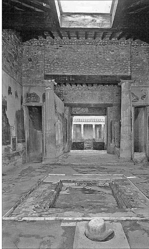
Figure 1.5 Atrium of a large house in Pompeii. Roof rainwater was directed into the basin in the center, from which it was directed into an underground cistern. Overflow was conveyed to the street (Photo V. Novotny).
