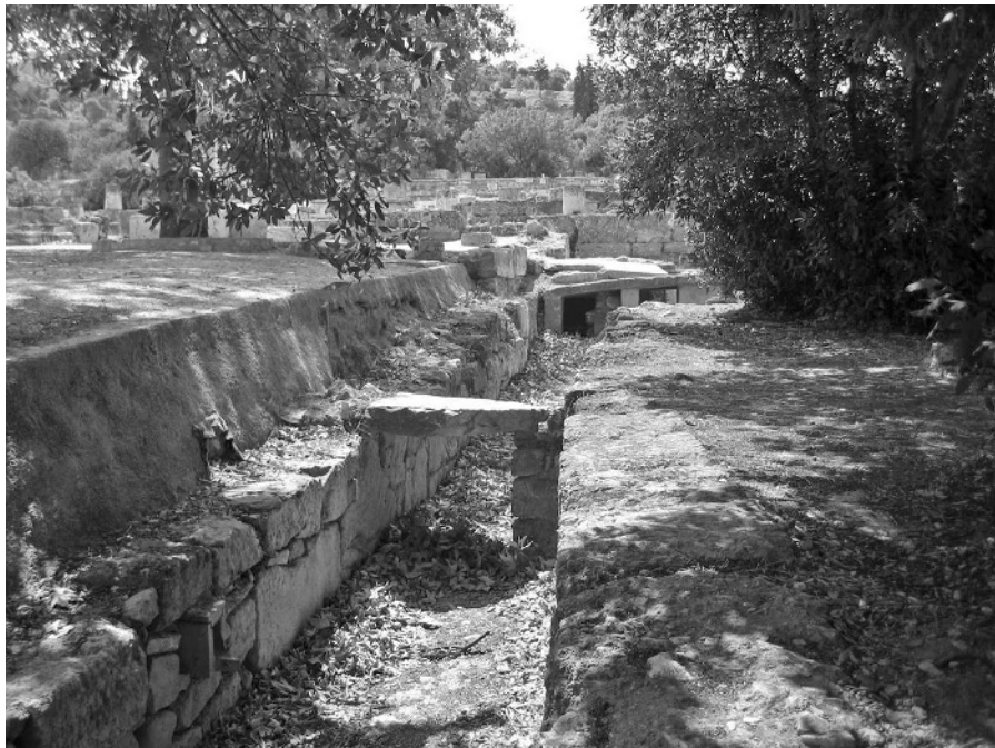
Figure 1.2 Drainage systems in ancient Athens (ca. 500 B.C.). This 1 m x 1 m surface drainage channel is located in the agora (gathering place) of the ancient Greek metropolis (Photo V. Novotny).
