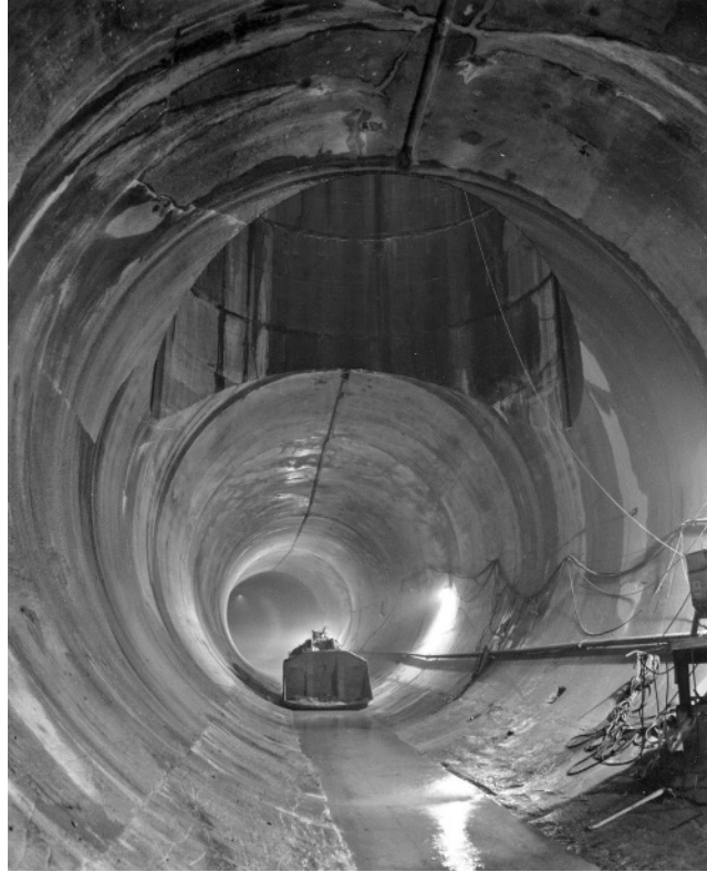
Figure 1.18 Deep tunnel storage of CSOs and SSOs in Milwaukee, Wisconsin. The stored mixture of rainwater and sewage is pumped for treatment. A similar but much larger tunnel system was excavated in Chicago, Illinois. Courtesy Milwaukee Metropolitan Sewerage District (MMSD).
