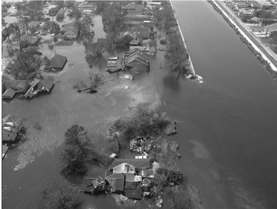
Figure 1.1 Impact of Hurricane Katrina in New Orleans (Louisiana) in 2005. Urban infrastructure and human response failed.
