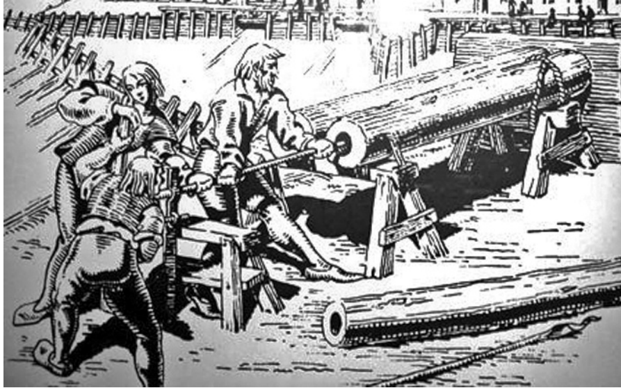
Figure 1.9 Making wood pipes for the medieval water supply systems (courtesy: Museum of Water Supply in Prague, Czech Republic).
