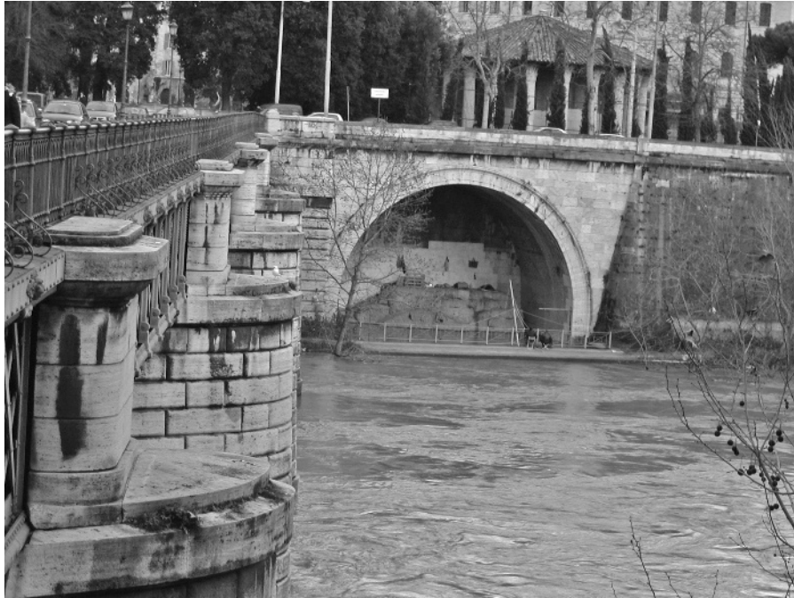
Figure 1.6 Outlet of the Roman sewer, the Cloaca Maxima (Largest Sewer) into the Tiber River. The sewer is functioning today, but a barrier was installed to prevent entry because of security concerns.
