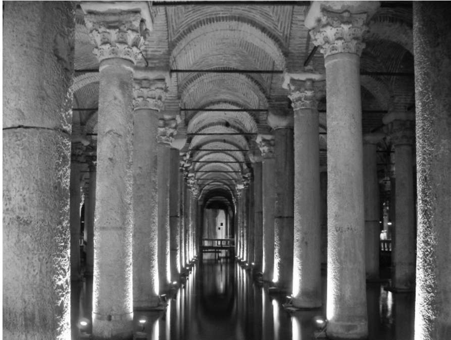
Figure 1.7 This underground Basilica cistern, capable of storing 80,000 m 3 (21.1 mg) of water, was built at the beginning of the seventh century in Constantinople, the capital of the Byzantine Empire (present-day Istanbul in Turkey) (photo V. Novotny).
