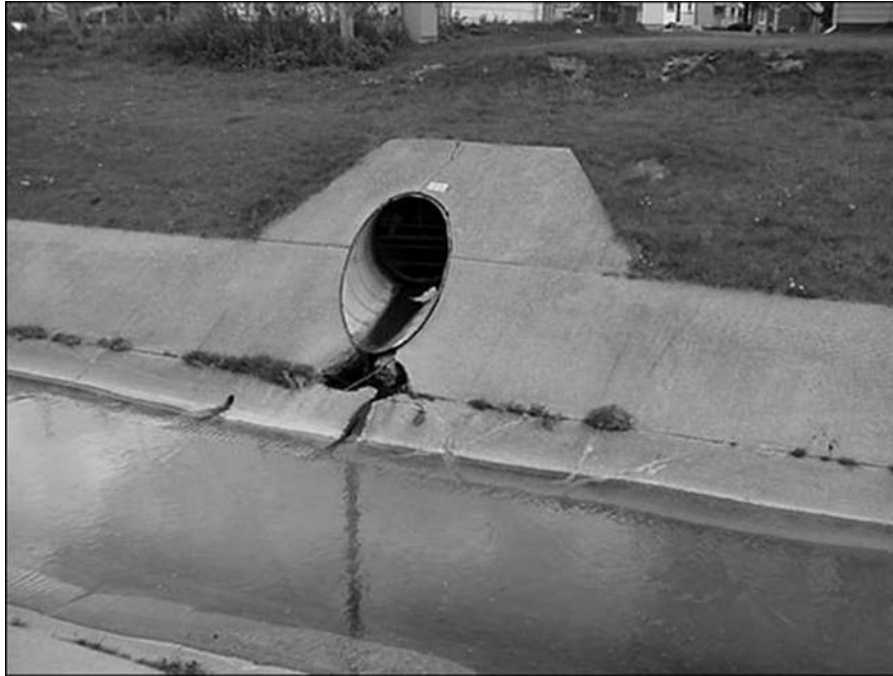
Figure 1.17 Lincoln Creek in Milwaukee, Wisconsin, was a concrete-lined channel receiving combined sewer overflows, before restoration in the 1990s. Photo V. Novotny.
