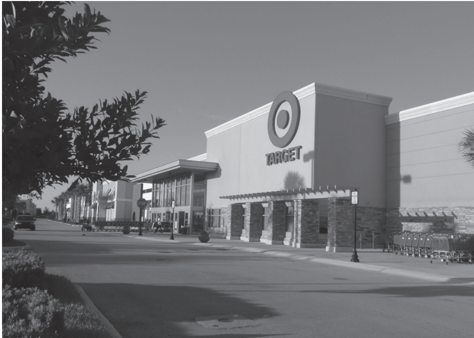
Figure 1-6 Community centers typically range from 250,000 to 350,000 square feet and are anchored with large-format discount department or home improvement stores. The centers also include multiple junior anchors such as apparel, arts and crafts, office supplies, shoes, and sporting goods stores. Gibbs Planning Group, Inc.
