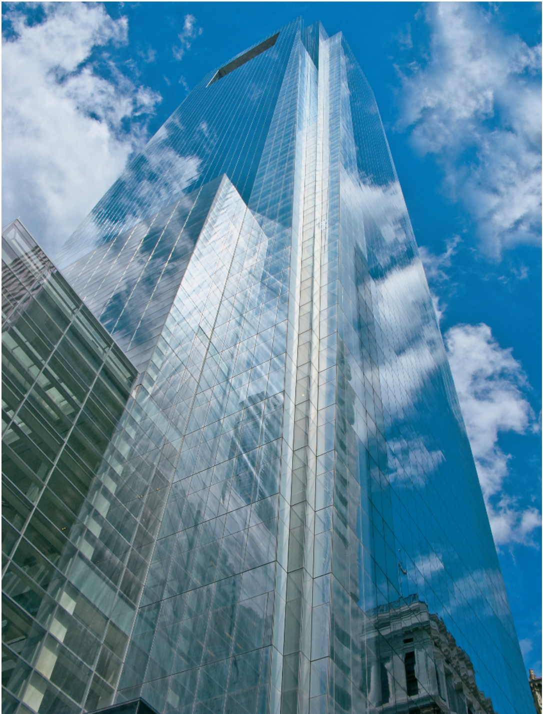
FIGURE 1.1 Comcast Center, Philadelphia, 2008, Robert A.M. Stern architect.
