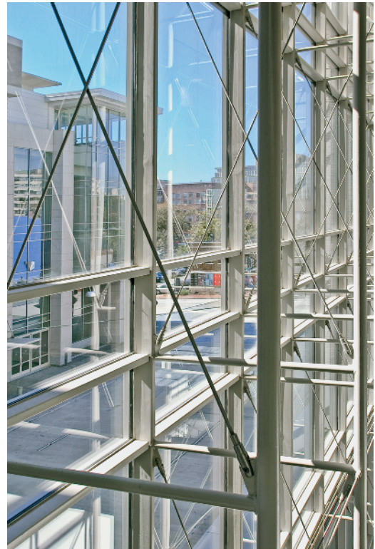
FIGURE 1.3 The Walter E. Washington Convention Center in Washington, D.C., 2003, is enclosed by an exposed truss system supporting an off-the-shelf stick curtain wall system. TVS-D&P-Mariani, PLLC JV architects.
