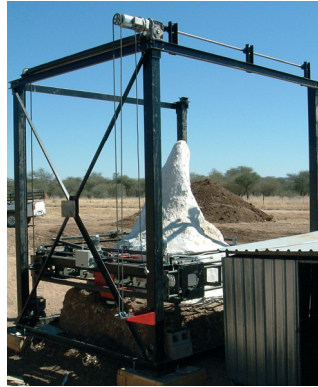
As part of the Freeform Construction research project at Loughborough University, the morphology of a Macrotermes michaelseni termite mound is scanned. See 'Manufacturing Performance' on page 42.
