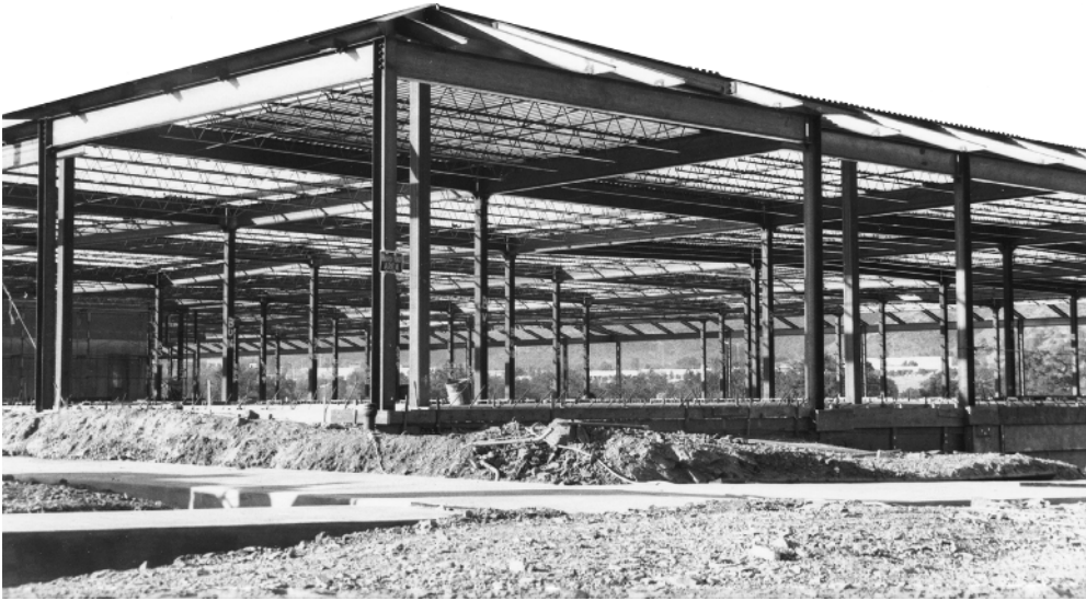
Figure 1.10 Two-way multiplication of structural units in a single-story building. The structure is achieved here at a medium scale with a common system: steel posts and beams, light steel truss rafters, and a light-gauge formed sheet steel deck.
