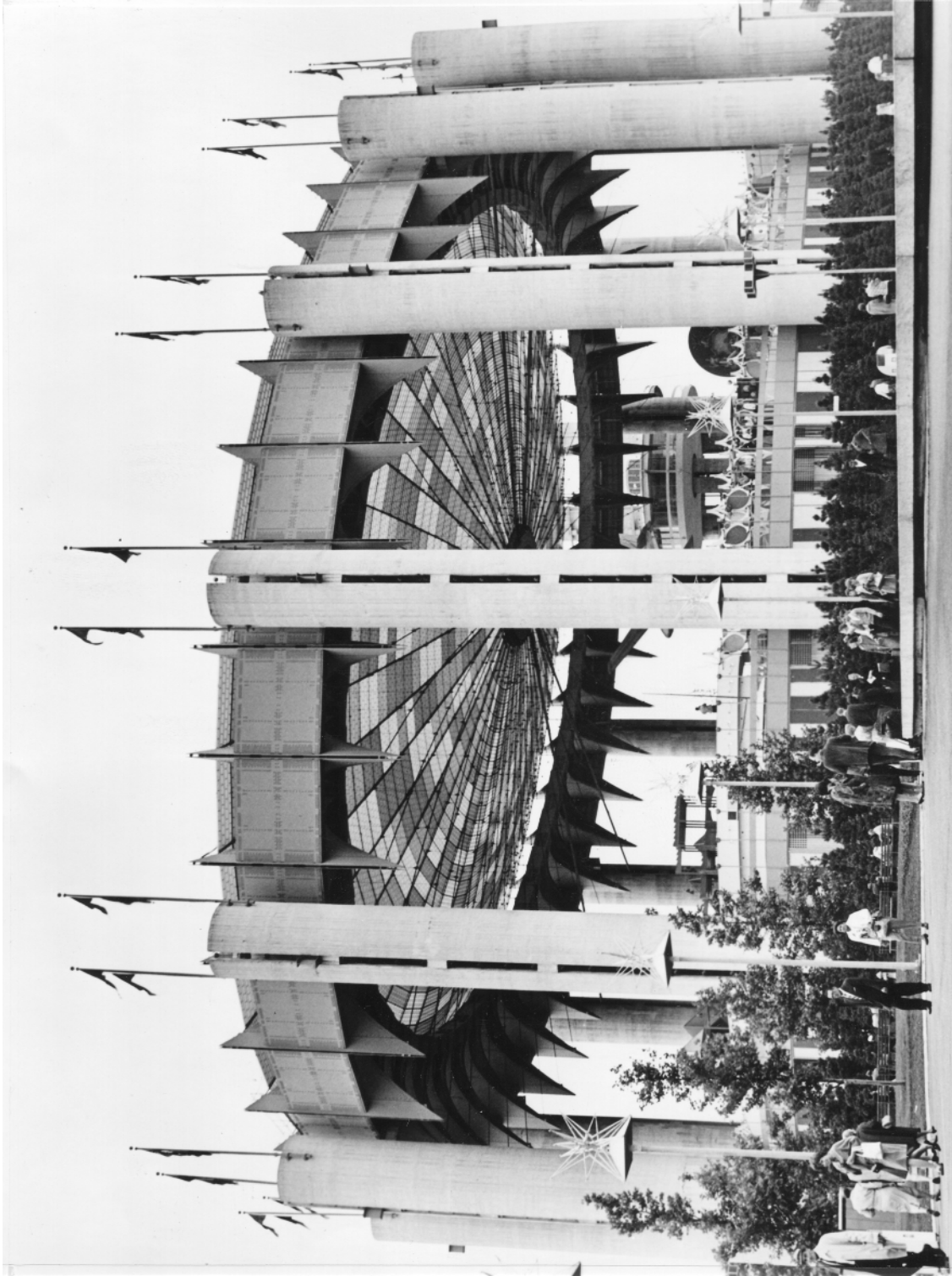
Figure 1.42 New York State's "Tent of Tomorrow" pavilion at the 1964 World's Fair. The 100-ft-high concrete columns carry an elliptical steel compression ring 350 \times 250 ft in plan. Suspended from the ring, a double layer of steel cables converges toward a steel tension ring at the center. The roof surface consists of translucent sandwich panels formed with two sheets of reinforced plastic separated by an aluminum grid. The panels, approximately 3000 in number, are trapezoidal in shape.
