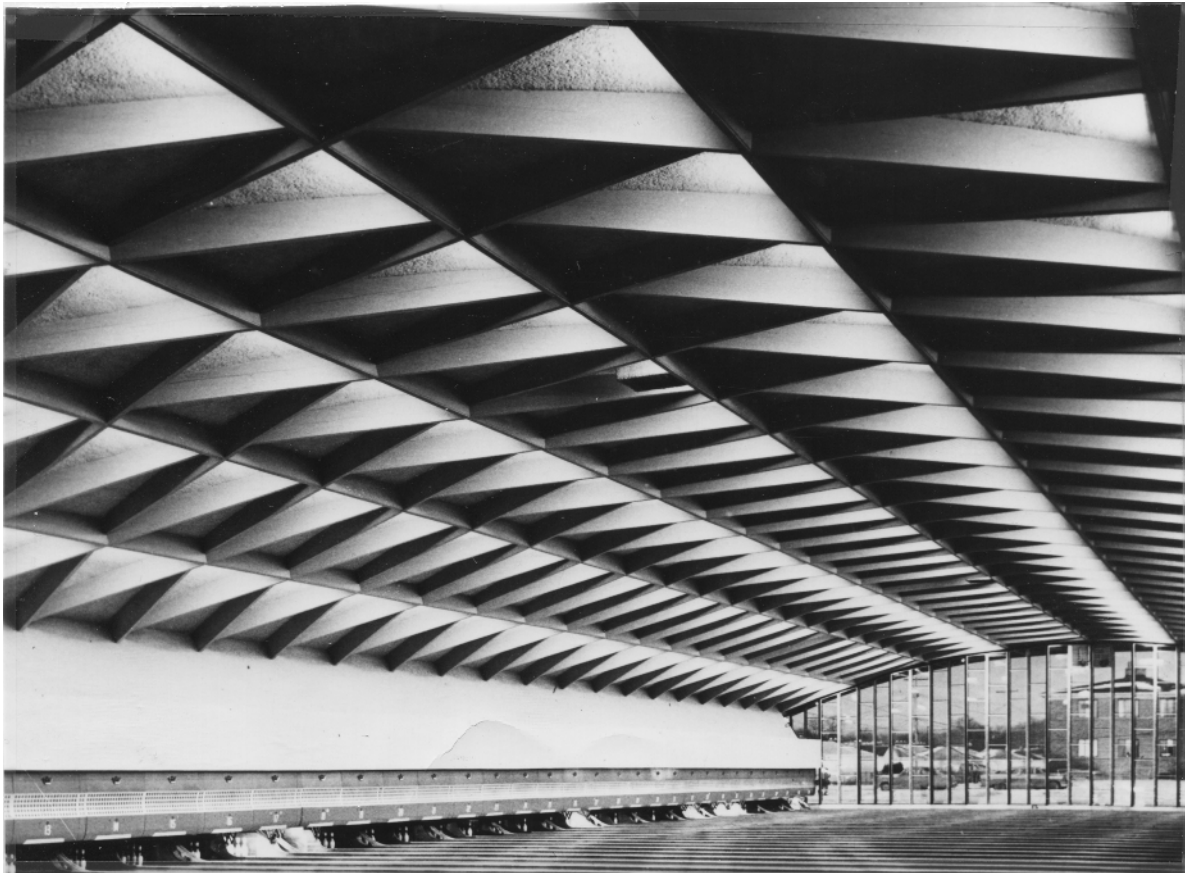
Figure 1.45 Wood lamella structure. Simple wood elements in a diagonal lamella pattern form this roof for a bowling alley.
