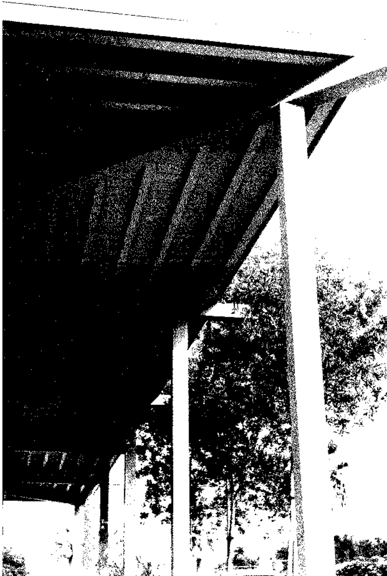
Figure 1.30 Simply detailed wood framing produces a structure with a clear lineage of historical development. Close inspection, however, reveals quite evidently that the elements are of contemporary industrialized origin, as opposed to the rough-hewn elements seen in Figure 1.25.
