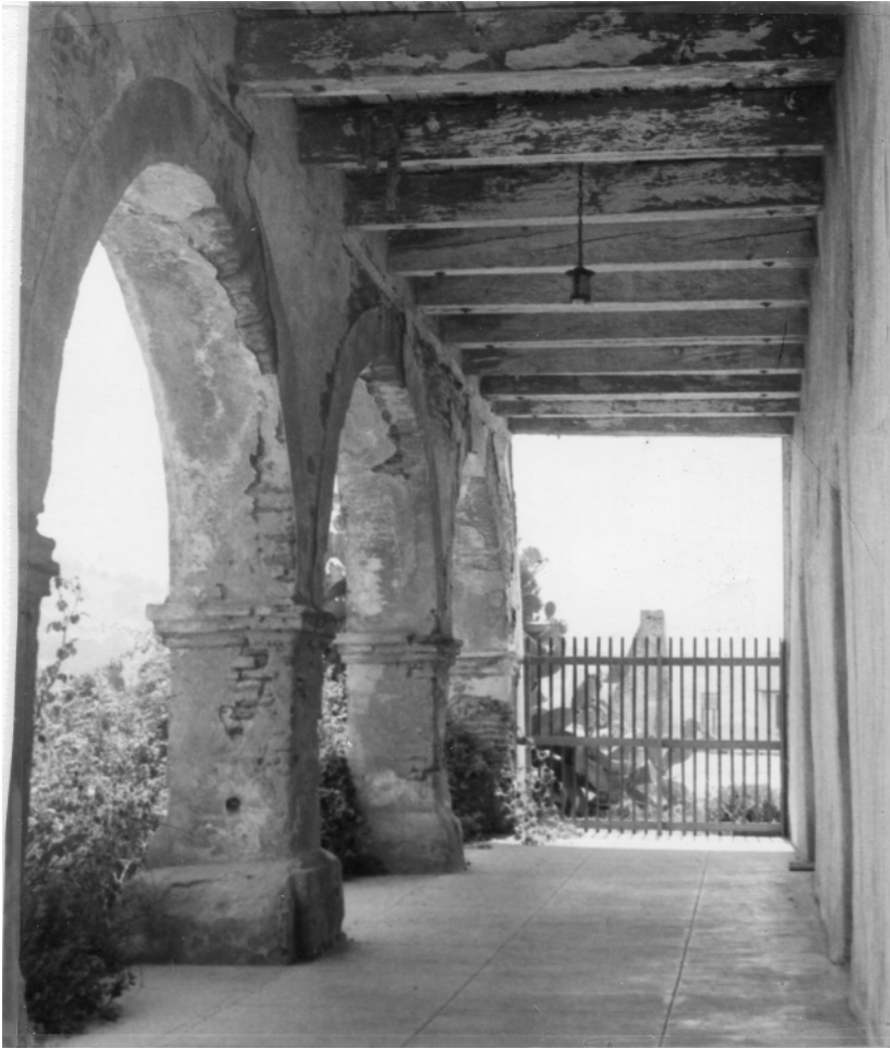
Figure 1.25 Historic construction with hand-hewn timbers and adobe brick walls and arcades.
