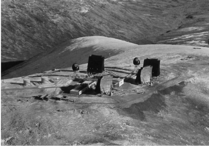
FIGURE 1.1 “White Alice” tropospheric communications site. (Courtesy of Western Electric.)
