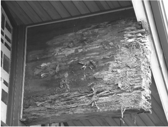
Figure 1.5.1-1 Advanced decay of unprotected glulam beam.
