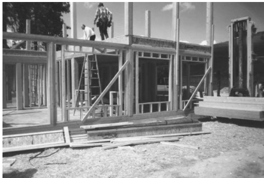
Figure 1.3.1-1 Post and beam construction.
