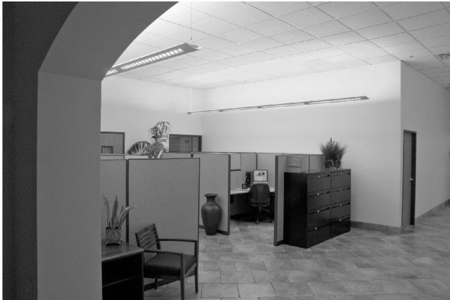
Figure 1-14b A lower mounting height improves the appearance and efficacy of indirect lighting systems. (Provided by Pinnacle Lighting.)
