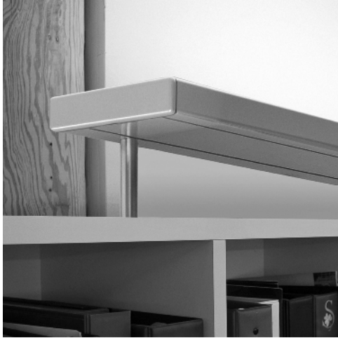
Figure 1-10 Use partition-mounted luminaires with white, reflective ceilings to provide soft indirect lighting without high installation costs. (Copyright the Lighting Quotient)
