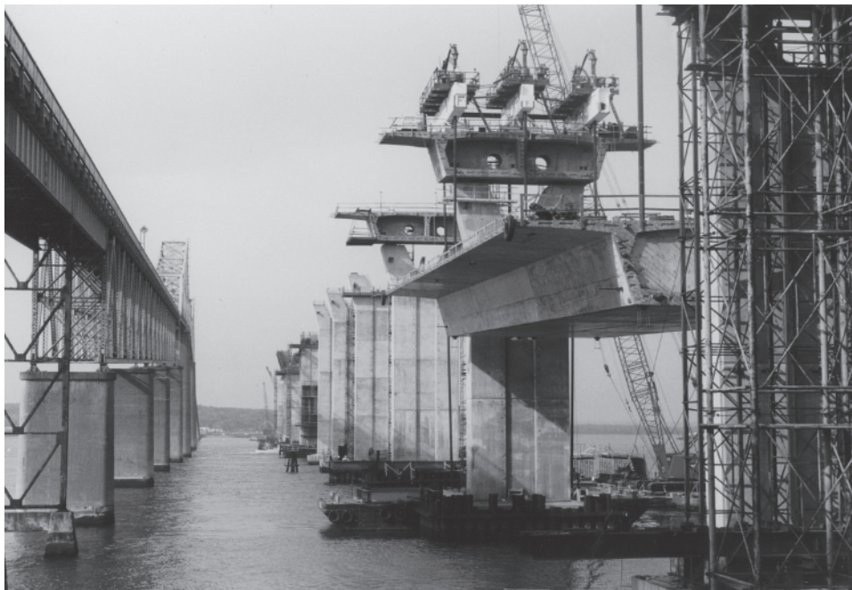
FIGURE 1.1 Prefabricated box girder deck being set in place. Courtesy of Michael Veech.
