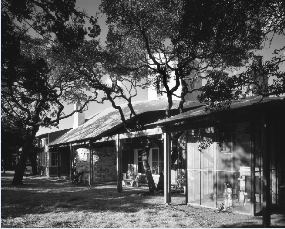
FIGURE 1.25 The curved roof shelters conditioned, enclosed, and open spaces, and is peeled back to admit mature live oak trees. 3D modeling the complex geometry resulting from the interaction of curved forms was more direct and accurate than constructing 2D drawings.
