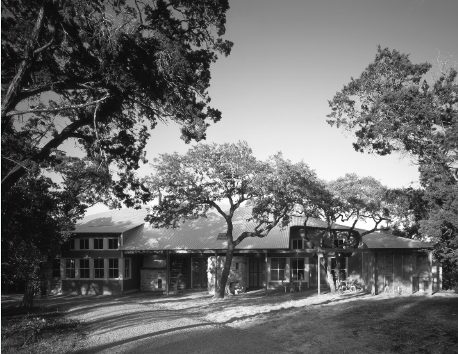
FIGURE 1.21 The project seen from the south. The roof's curved ridge and level perimeter created a complex curved surface that was more readily analyzed and represented with BIM. Note a portion of the original cabin visible behind the ladder, well-protected by the generous roof overhang.
