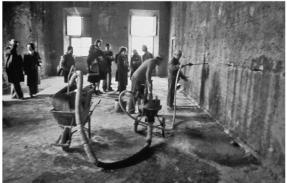
Figure 1-8 Cement grout injection during a 1977 restoration as a structural stabilization measure at the Ospedale di San Michele complex in Trastevere, Rome, is illustrative of one of several conservation-engineering techniques developed in Italy.
