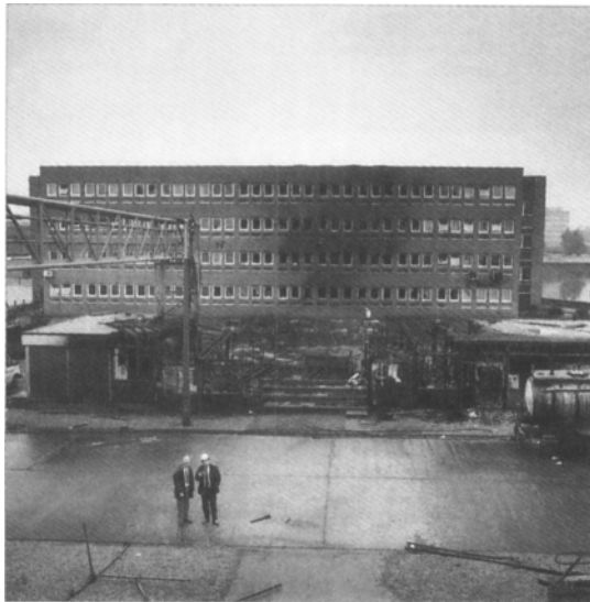
Figure 1.13. Damage to the Control Room and Impact on the Office Block from the Jet Flame at Hickson & Welch
