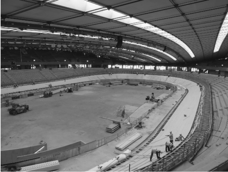
Some of the 56km of timber being installed to form the Velodrome's track (photo courtesy of Mark Lythaby).
