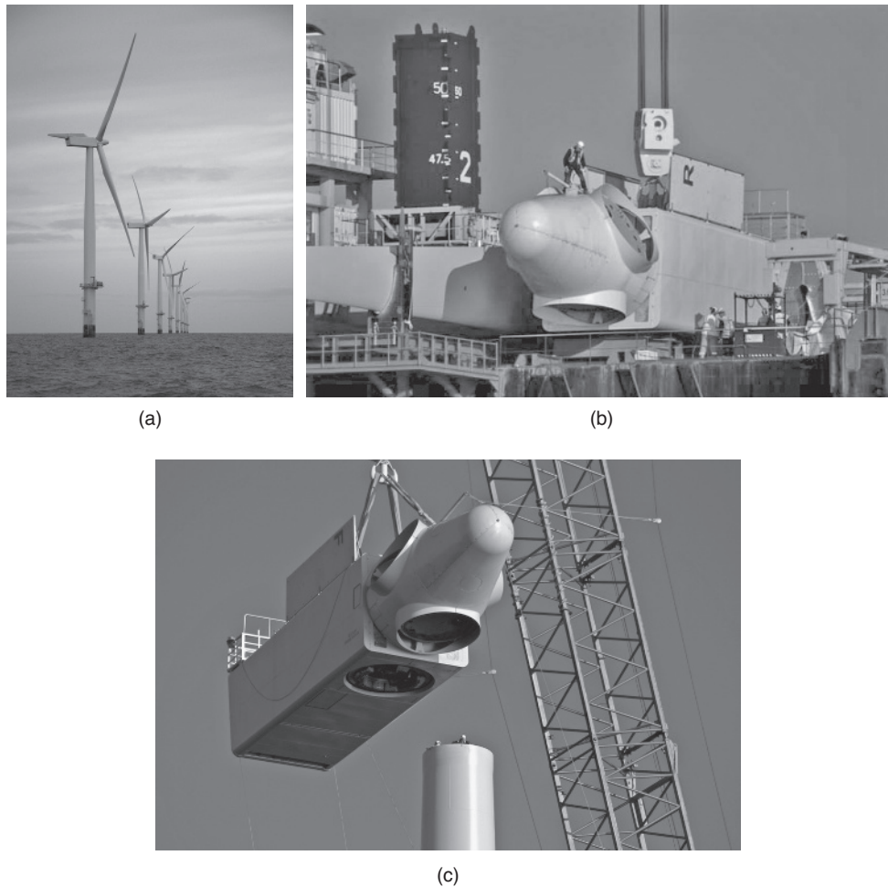
Figure 1.2 (a) Rhyl Flats Offshore Wind Farm. See Plate 1 for the colour figure. (b) 3.6 MW nacelle prior to lifting. (c) Assembly of 3.6 MW wind turbine. Rhyl Flats Offshore Wind Farm consists of 25 \times 3.6 MW Siemens wind turbines. Hub height – 80 m above mean sea level (MSL). Height to blade tip – 134 m above MSL. Rhyl Flats Offshore Wind Farm was built and is operated by RWE npower renewables. Photographer: Guy Woodland. Photos reproduced courtesy of RWE npower renewables. See Plate 2 for the colour figure
