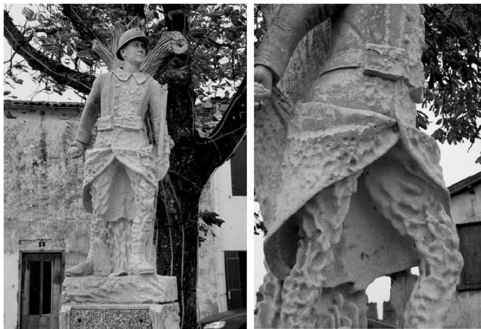
Figure 1.5 Day after day this statue has endured the endless deposit of salt-spray (courtesy of Leo Pel, Eindhoven University of Technology). The weathering results from the in-pore pressure buildup due to the crystallization of sea-salts induced by the drying following each deposit. For a quantitative analysis see Section 9.3.4
