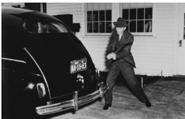
Figure 1.7 Henry Ford demonstrating the strength of the bioplastic car body. Courtesy of The Henry Ford
