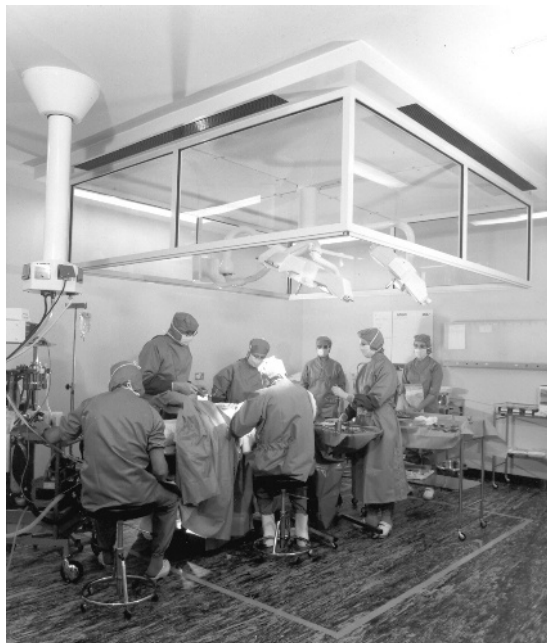
Figure 1.4 Unidirectional airflow system and occlusive clothing used in an operating room
