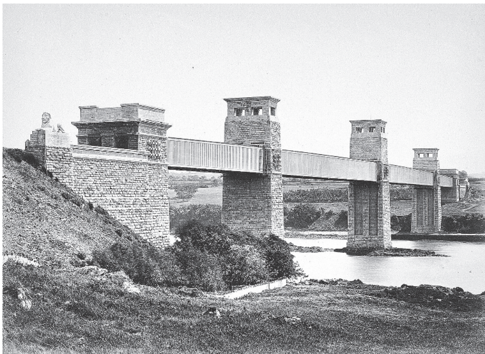
Figure 1.23 The Britannia Bridge, 1850, North Wales (Source: Courtesy of the Los Angeles County Museum of Art).
