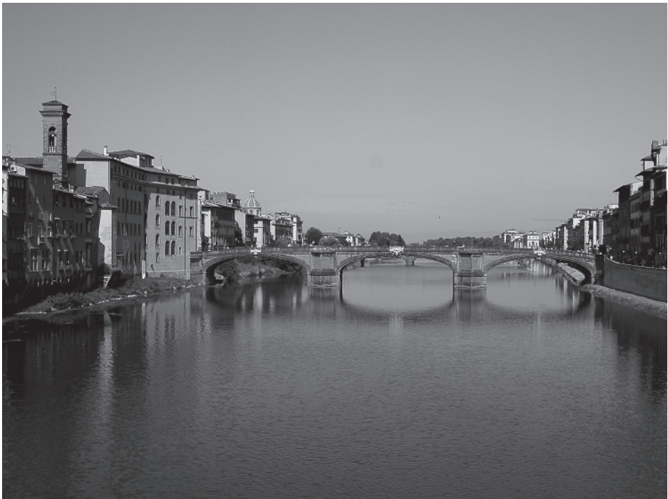
Figure 1.19 Santa Trinita Bridge in Florence, sixteenth century (Source: Photography by Bruno Barral/ https://commons.wikimedia.org ).
