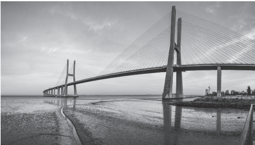
Figure 1.2 (a) The Öresund link between Sweden and Denmark, 2000 (Source: Soerfm, http://commons.wikimedia.org/wiki/File:Öresund_Bridge_-_Öresund_crop.jpg#mediaviewer/File:Öresund_Bridge_-_Öresund_crop.jpg , CC BY-SA 3.0.), and (b) the Vasco da Gama Bridge, in Lisbon, Portugal, 1998 (Source: Photograph by José Araujo).
