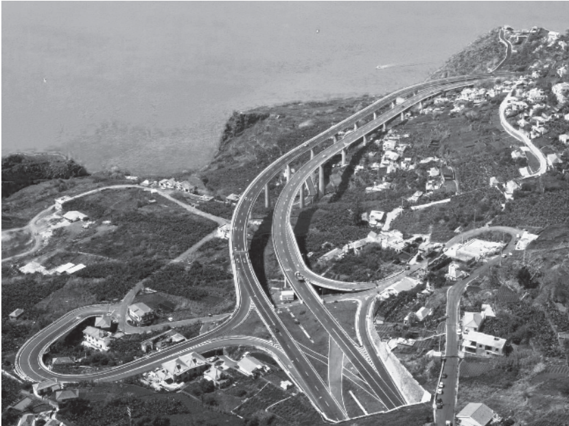
Figure 1.1 (a) The Freixo Bridge over the river Douro in Oporto, 1993, and (b) a viaduct in Madeira Island, Portugal, 1997 (Source: Courtesy GRID, SA).
