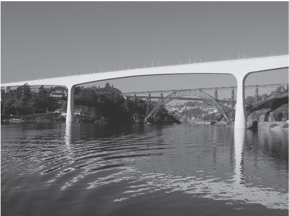
Figure 1.31 The São João Railway Bridge, 1990, Oporto, Portugal (Source: Photograph by Joseolgon/ https://commons.wikimedia.org / Public Domain).
