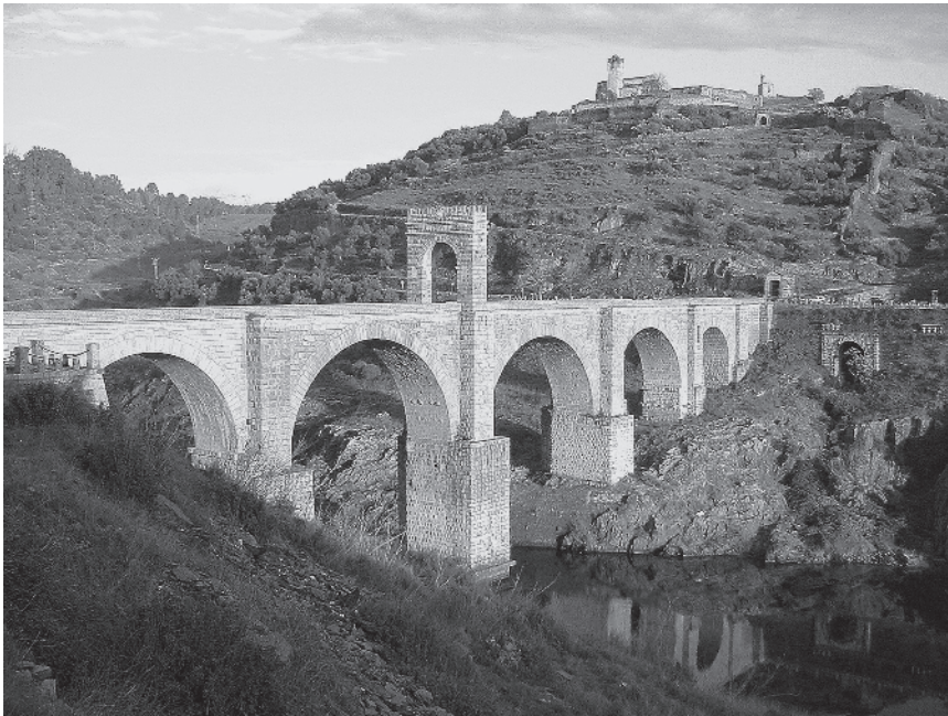
Figure 1.18 The Roman Alcantara Bridge in Spain, second century (Source: Photography by Dantla/ https://commons.wikimedia.org ).
