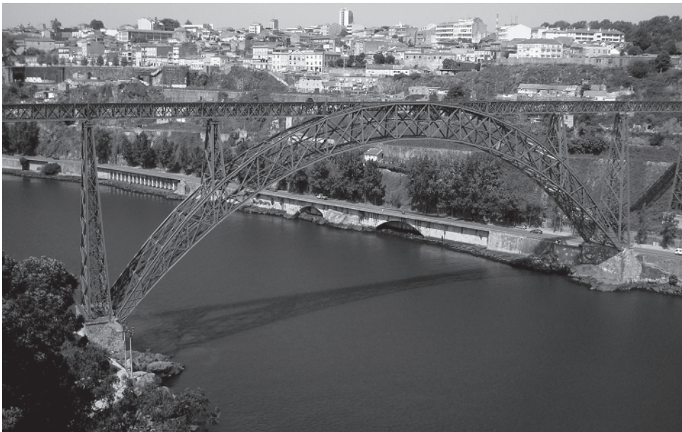
Figure 1.24 Maria Pia Bridge, 1877, Oporto, Portugal (Source: Photograph by José O. Pedro).
