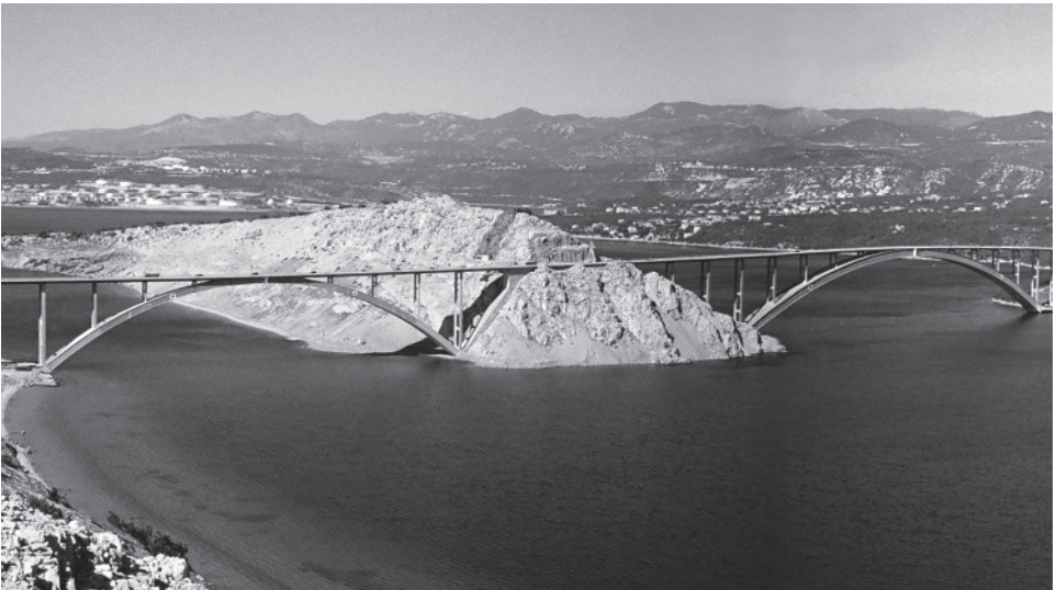
Figure 1.29 The Krk reinforced concrete arch bridge, 1979, former Yugoslavia (Source: Photograph by Zoran Knez/ https://commons.wikimedia.org ).
