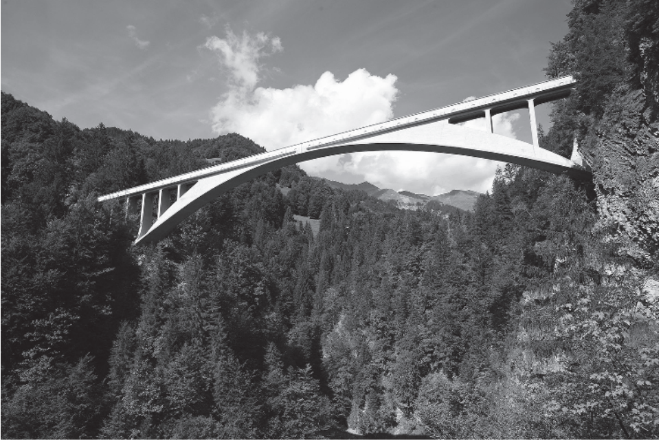
Figure 1.28 The Salginatobel Bridge, 1930, Switzerland (Source: Photograph by Rama, https://commons.wikimedia.org/wiki/File:Salginatobel_Bridge_mg_4077.jpg . CC BY-SA 2.0 FR).
