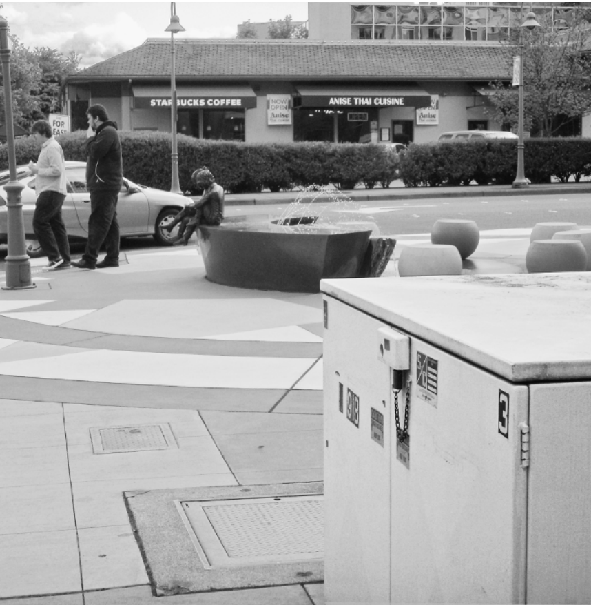
Figure 1-20 Utility boxes should be placed with pedestrian access and public spaces in mind to avoid unfortunate consequences for streetscape designs.
