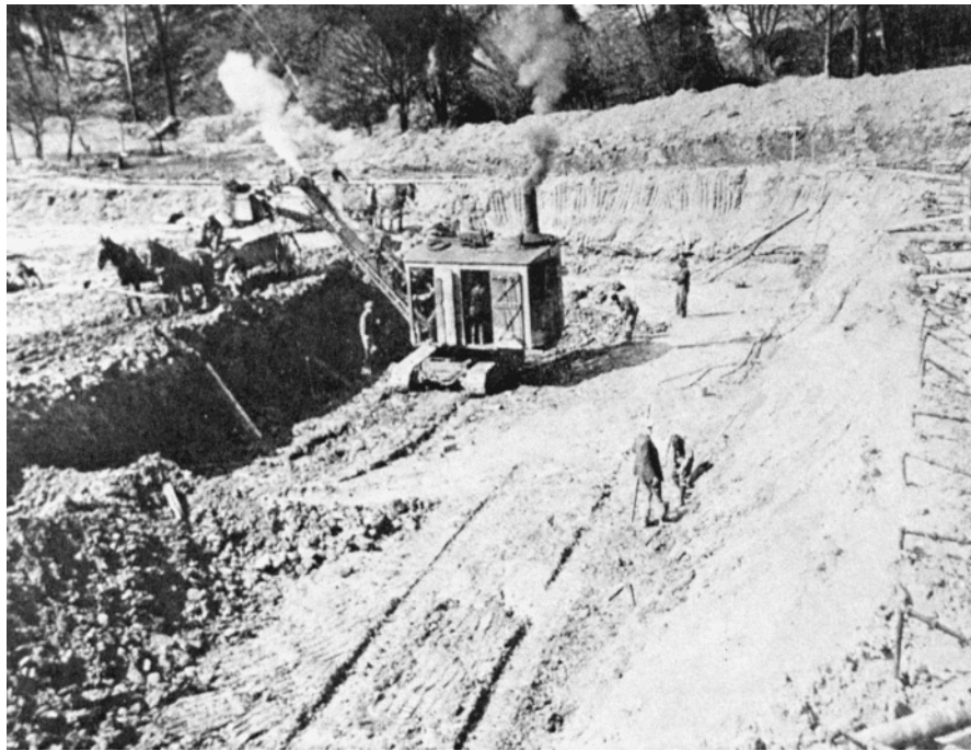
Figure 1.4 An early wellpoint system (c. 1928). Courtesy Moretrench.
