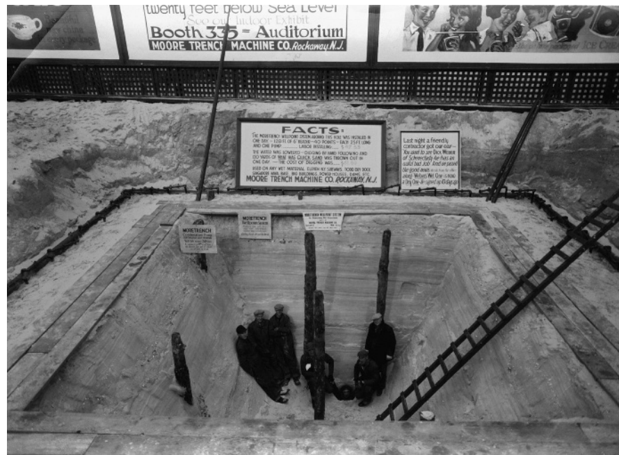
Figure 1.5 In 1930, Moretrench demonstrated the use of wellpoints at the Road Show in Atlantic City, New Jersey, lowering the water table next to the Boardwalk by 22 ft (6.7 m). Courtesy Moretrench.
