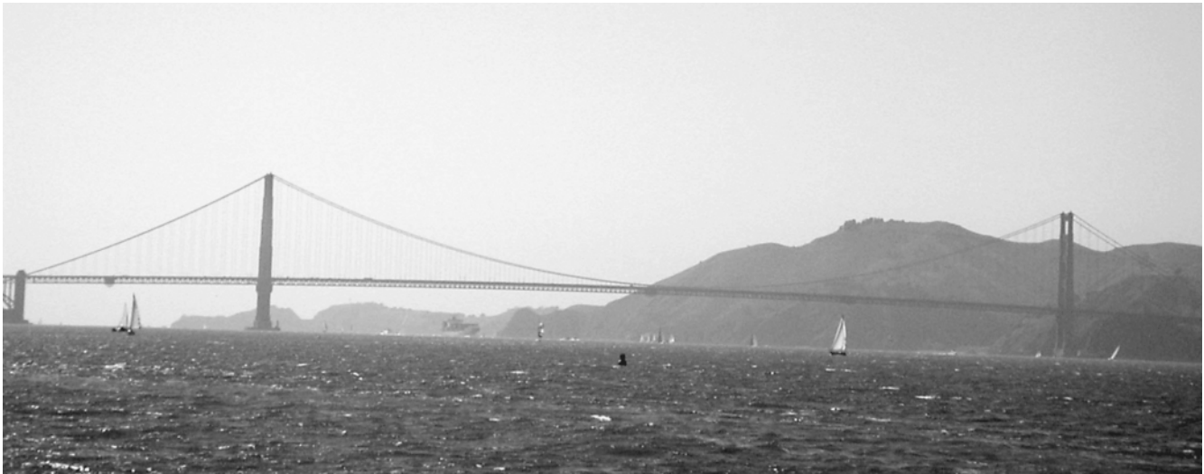
Figure 1.28 The Golden Gate Bridge.
