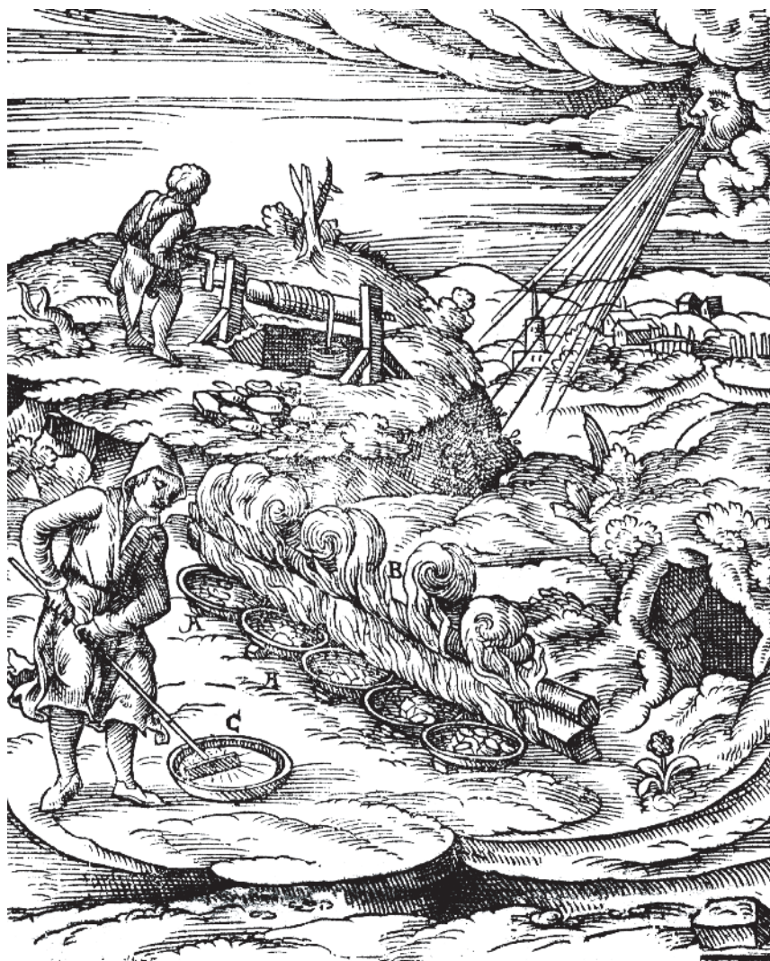
FIGURE 15. ■ Smelting of bismuth ore in open wind; freshly formed molten bismuth flows into the pans (Ercker, see Figure 5).
